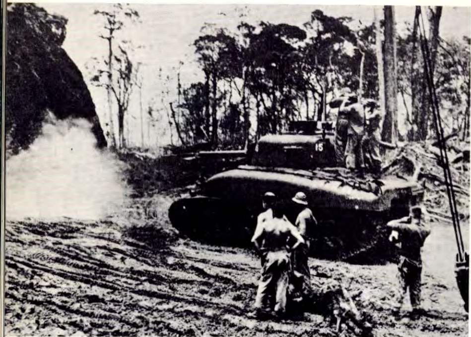
Drilling blast holes with a tank gun speeded road building
