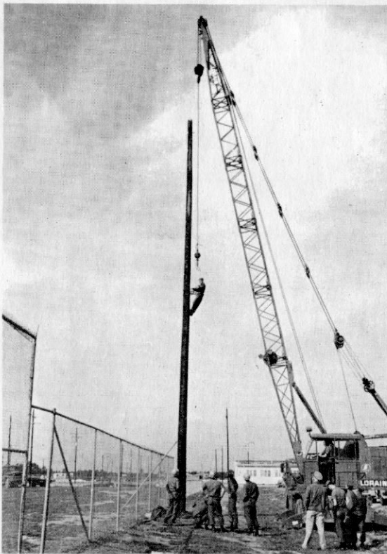
CBC BALL FIELD — Equipment Operator First Class E. D. Graves operates the crane while Construction Electrician Third Class W. M. Myers removes sling from pole which will support lights for night games.
