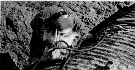
GULFPORT ROAD PROJECT — Steelworker Third Class W. Reichardt welds a flange on a culvert.
