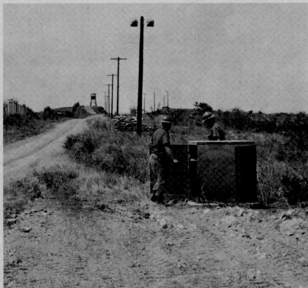
LOOKS GOOD--LT(jg) Louis F. Campbell, Officer in Charge of Detail GITMO, and Chief Builder Billie H. Newman inspect a terminal box on the security fence lighting project.
