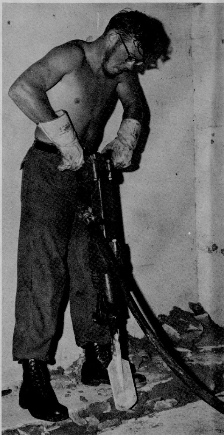
HAMMERING --Utilities Man Third Class K. E. Norton uses a pneumatic hammer to break up cement floor so a new sewer line can be installed in Fajardo's future recreation center for the aged. Like his co-workers, PO3 Norton is assigned to Bravo Company with NMCB-62.
