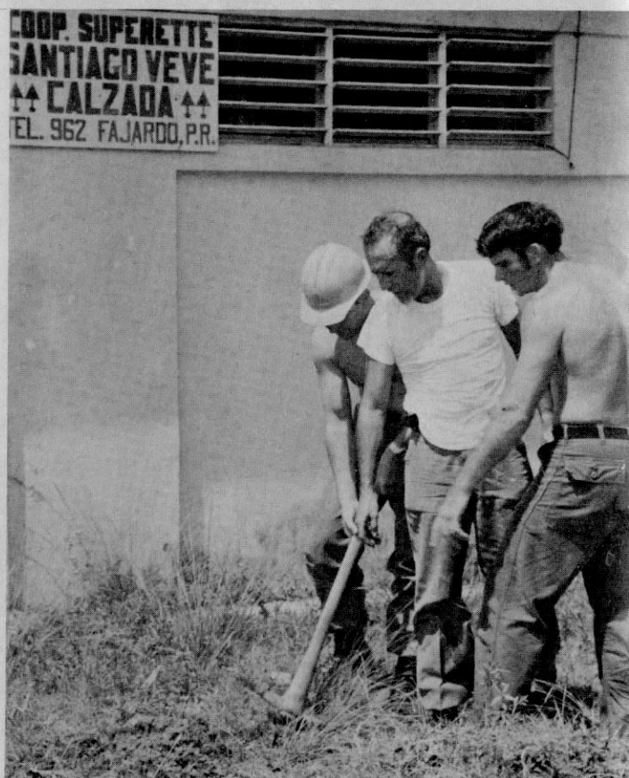
DIGGING IN-Lieutenant (j.g.) G.D. Hagedorn uses a pick to break ground near old water line so it can be taken and replaced. Utilities Men P. R. Hagedorn and C. H. Owenby discuss the operation.
