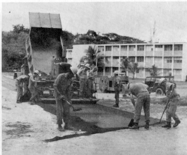
Alfa Co. personnel lay an asphalt driveway at the Bundy BEQ.
