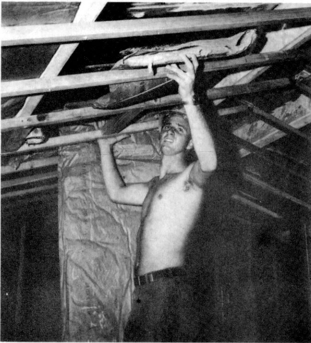
BU3 St. Jean works on the hospital addition, insulating the roof of the butler building.
