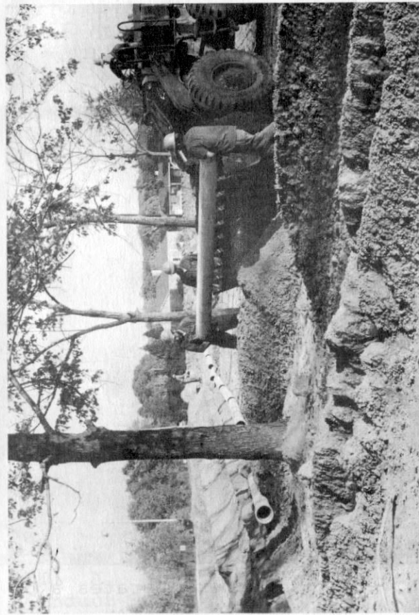
Workers place sewer pipe for the trailer park.
