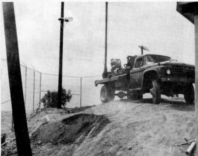
CE's maneuver an auger truck into place to drill pole holes for the security lighting project.
