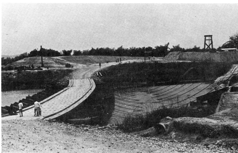
BRIDGE PROJECT -- A temporary pontoon bridge spans the Cam Lo River. MCB 62 is building a permanent bridge to replace it. The first pile for the new bridge is at the left of the picture, and wreckage of an old one is at the right.
