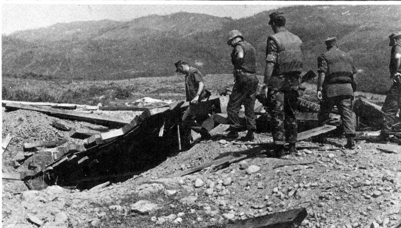
BLOWN -- A survey party inspects the remains of bridge 910, blown apart by satchel charges early in the morning of April 20. MCB 62 rebuilt the structure in only three days. (See story -- Page 1)
