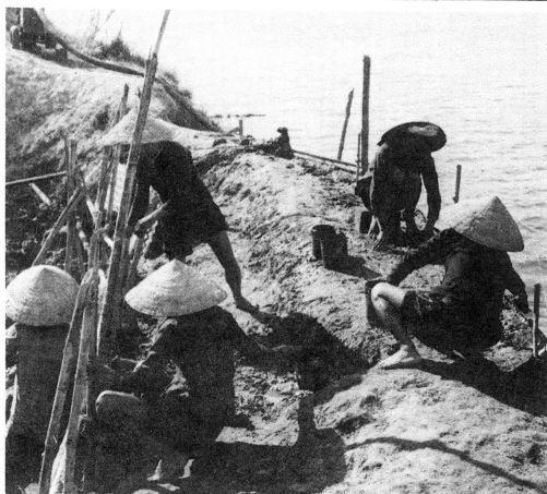
VIETNAMESE GIVE A DAM -- Vietnamese workers construct a cofferdam at the Cam Vu pumping station. 62's Civic Action Team enlisted their aid in the repair of the station.
