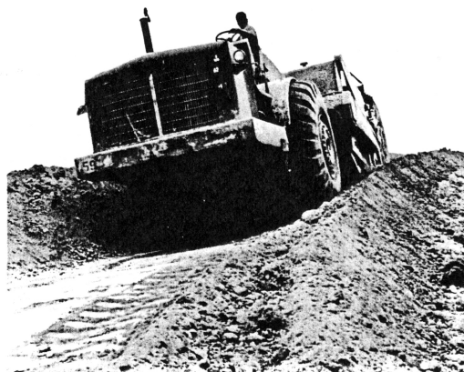
FILL 'ER UP -- An equipment operator loads his scraper with dirt to be used as fill material along the highway.
