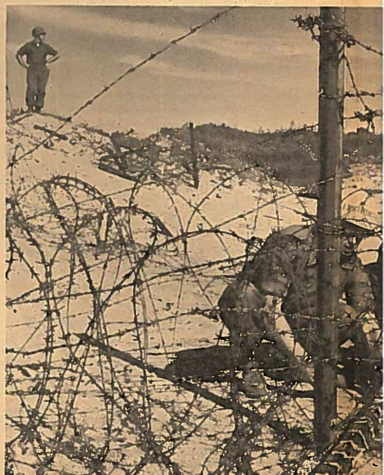
Construction Apprentice Richard Bonilla places an improvised "Bangalore Torpedo" charge under the guidance of his clear
