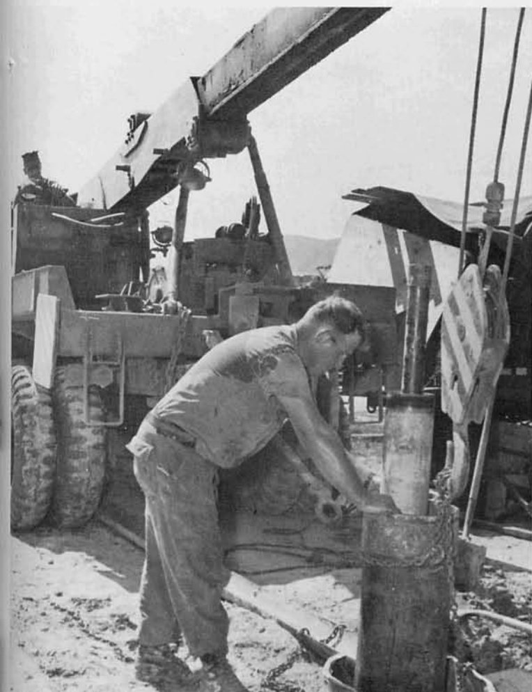
Pulling surface casing
