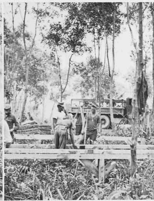
0900: Jacks for the CAC Team huts are positioned.
