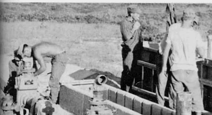
Installing the new Pumps for the Phu Bai Water System.
