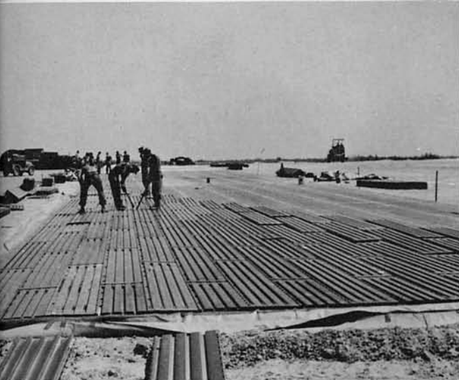
Laying the matting for 6 acre Helicopter Parking Apron
