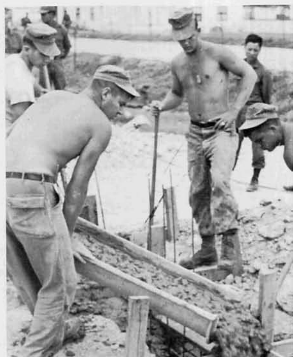
Placing foundation—Hue Interrogation Center
