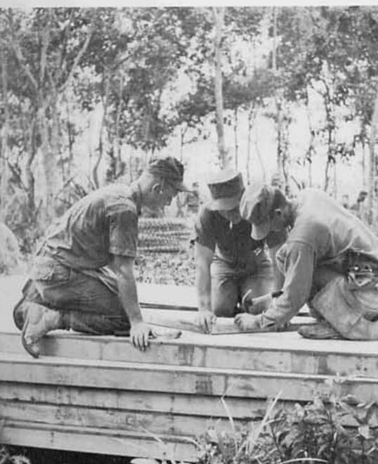
1000: Deck sections are prepared for quick installation.
