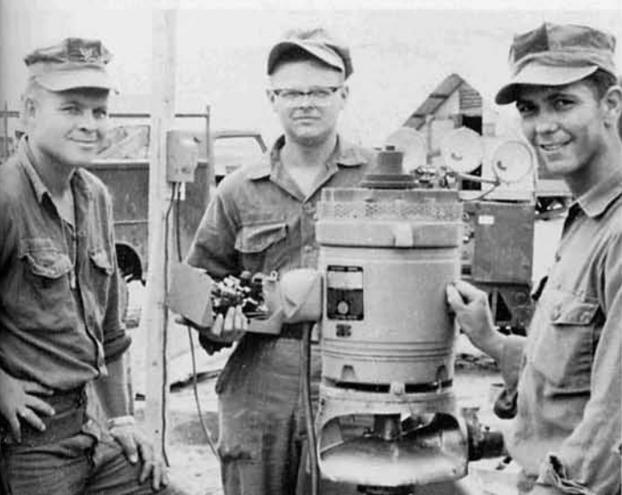
Setting motor controllers on well pump
