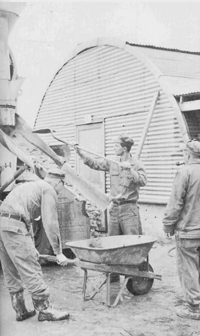
Concrete batched at the plant was used throughout the Combat Base and surrounding areas
