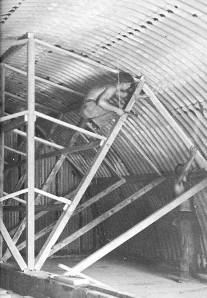
Shoring an ammo bunker at ASP-2.
