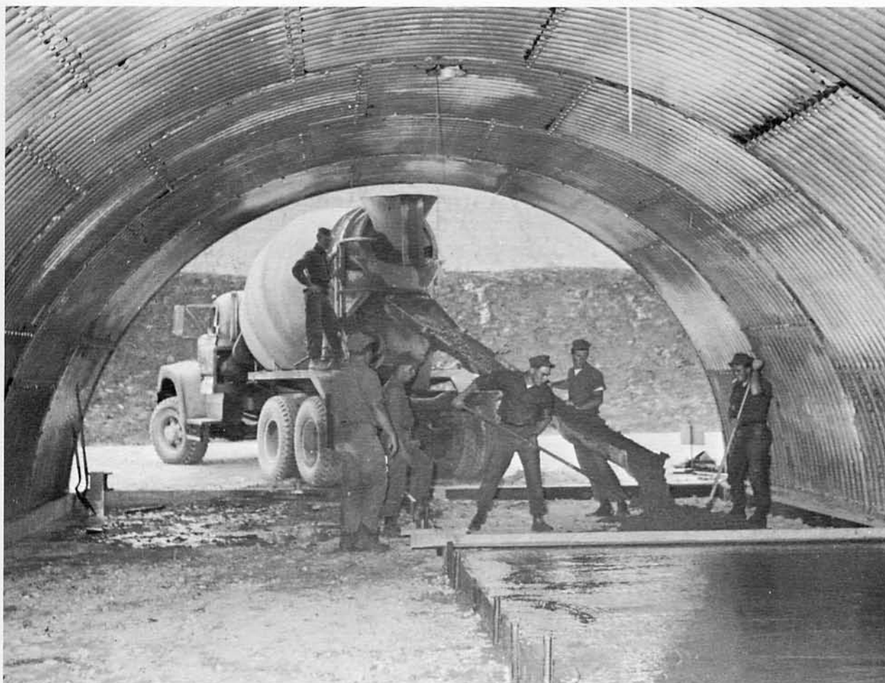
Delta pours the pad for an ammunition bunker at Ammunition Supply Point #2.
