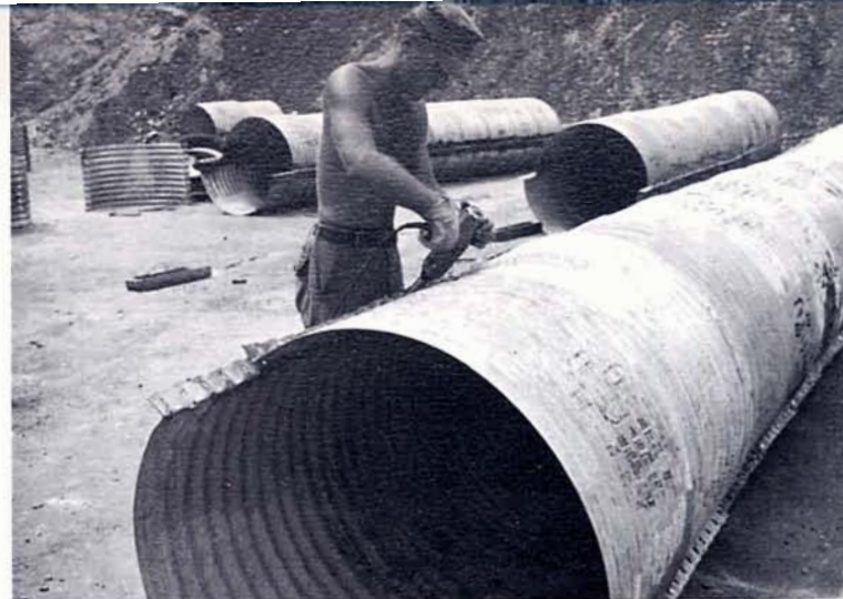
Delta workers fabricated and installed culverts.
