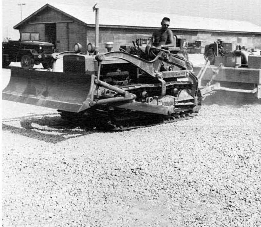
Right: EO3 Howard P. Boehme compacts gravel at the first Light Anti-Aircraft Missile Battalion parking lot. Below: MR2 Gary Purdue at work in Alfa's machinery repair shop. Lower right: 62 SEABEES work with Marines to clear a defensive perimeter near Danang.
