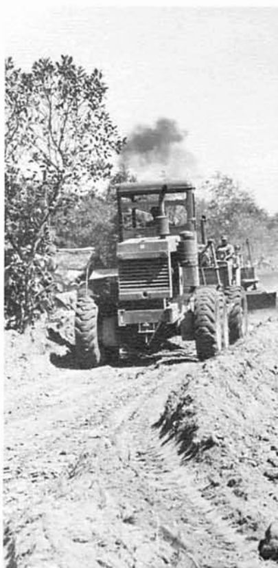
Above: MCB 62 Equipment Operators level fill dirt on highway #1 near Phu Bai. Left: Donald E. Rouse, EO2, cleans a discharge chute on MCB 133's asphalt plant. The Phu Bai detail worked with MCB 133 and other Battalions to upgrade route #1.
