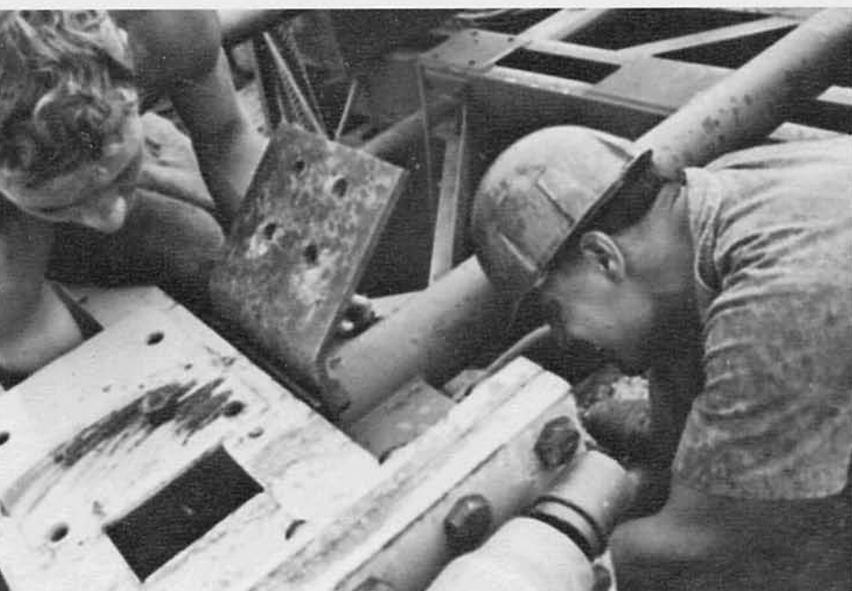
Above: SW3 Robert Porter and SW2 William Steffen assemble trestles for the Dong Ha Bridge. Right: SW3 Leo Boeding welds a wire cage used to enclose the bridge trestles. Opposite page, left: SW2 Steffen and CN Gary Russell tighten bolted joints on the bridge. Opposite page, right: BU2 Kenneth Struewing, BU3 Daniel Griffith and BU3 Gregory Mascio set steel plates over pile cap anchor bolts.
