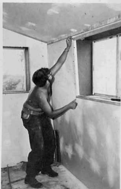
BU3 Kell at the Hospital Addition
