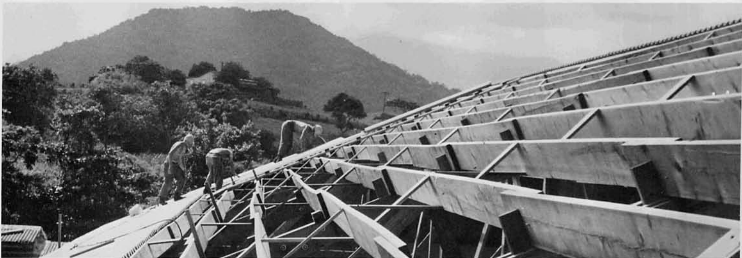
Delta Company Builders installing roofing on the Navy Exchange Warehouse
