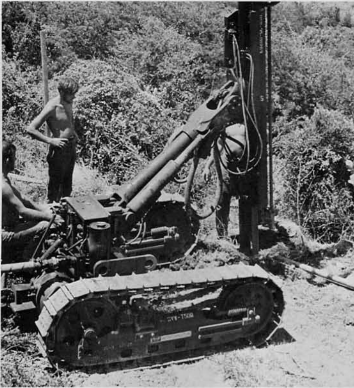
SW2 W. L. Mathis drills a hole for a fence post.
