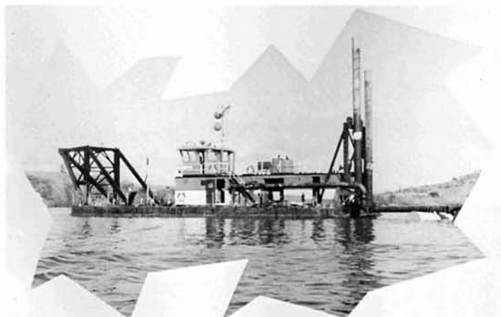
Dredging work at Guantanamo Bay. Not pictured is Dredge SCPOIC Benjamin C. Wray
