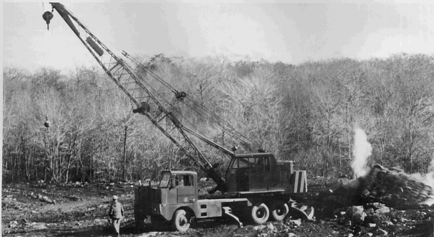
Blasting in New London
