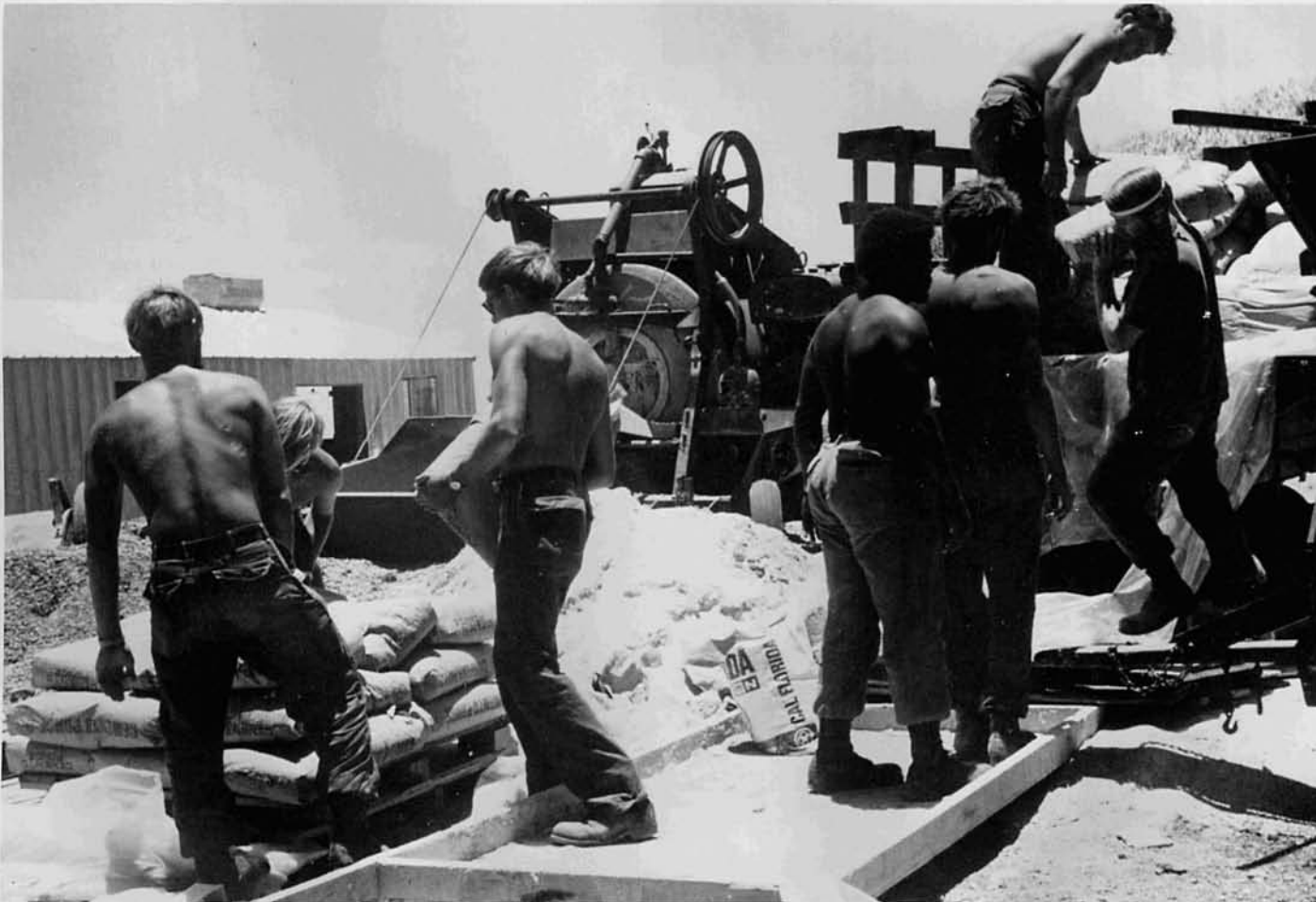
Detail members prepare for pouring concrete tank supports.
