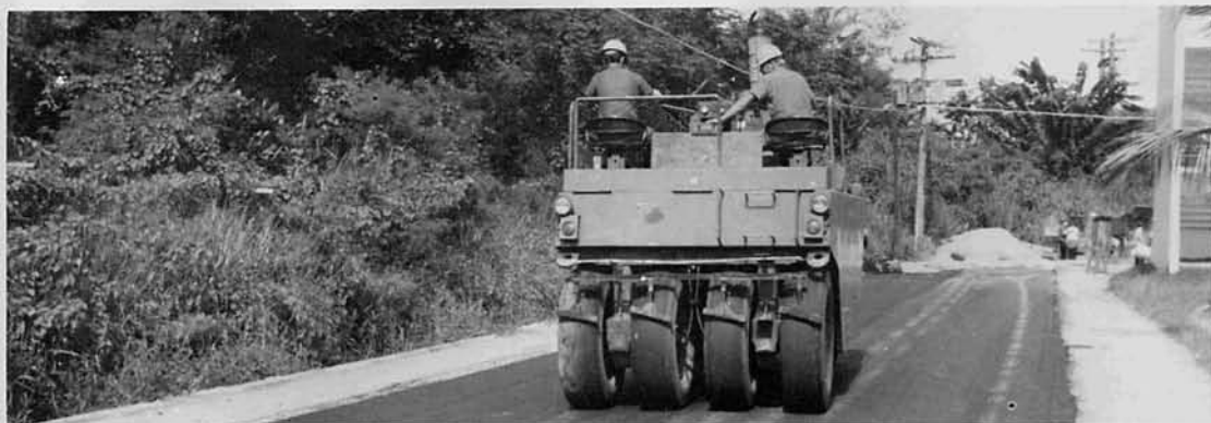
Rolling the pavement at Bundy
