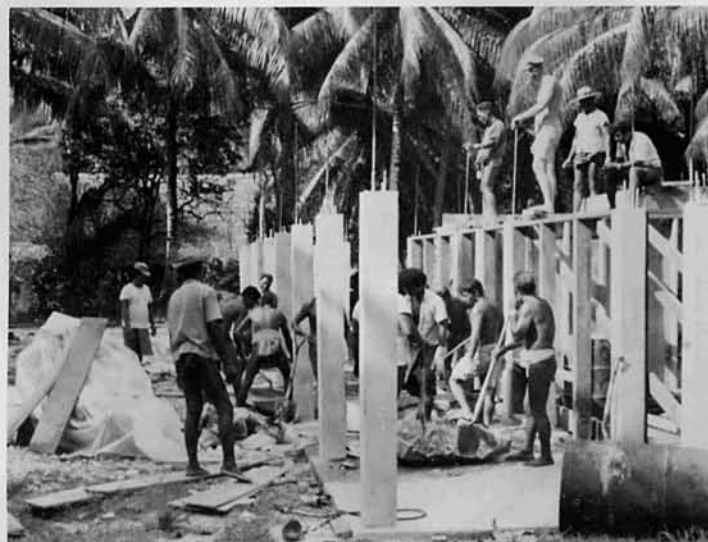
UT3 Richardson supervises the Lamotrek Islanders in mixing concrete for the water catchment in the dispensary.
