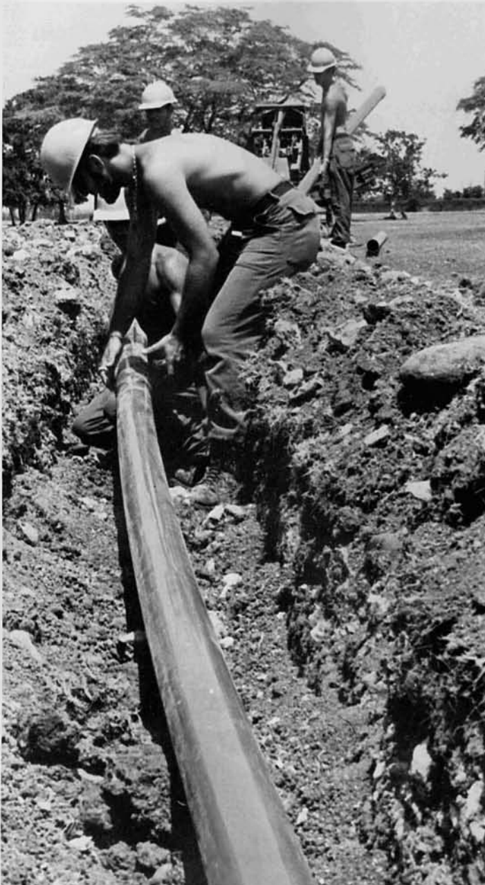
Irrigation work at Fort Allen
