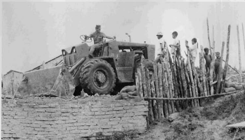
Leveling and compacting the access road to the Cham village in Ham Tan.
