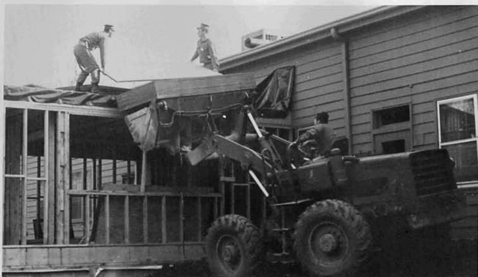
Unloading Plywood roofing
