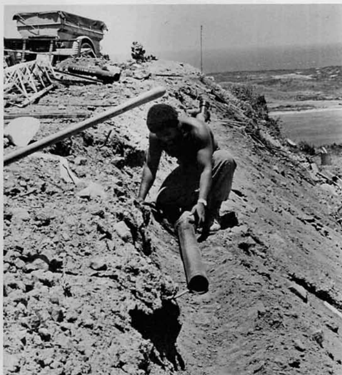
UT3 Ralph Copeland places a section of sewer pipe at the observation point.
