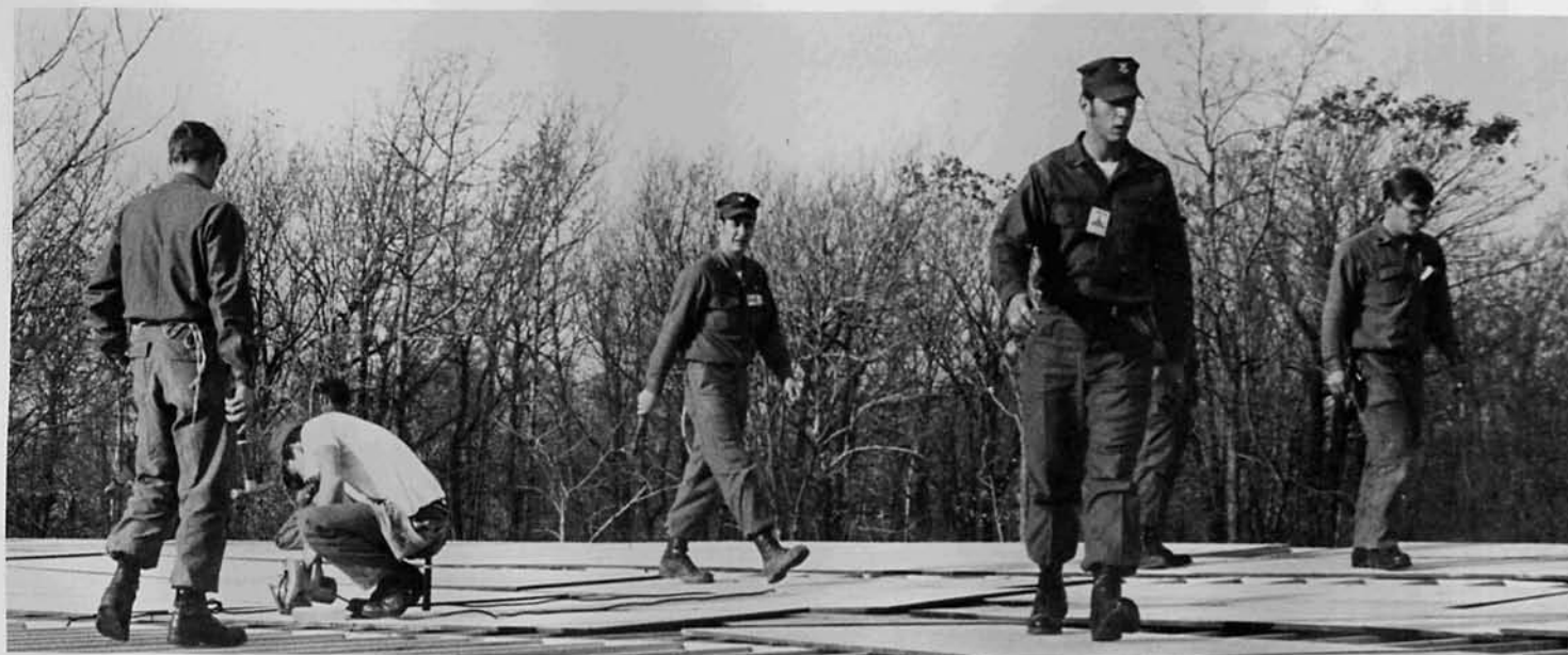
Top deck of the staff support facility
