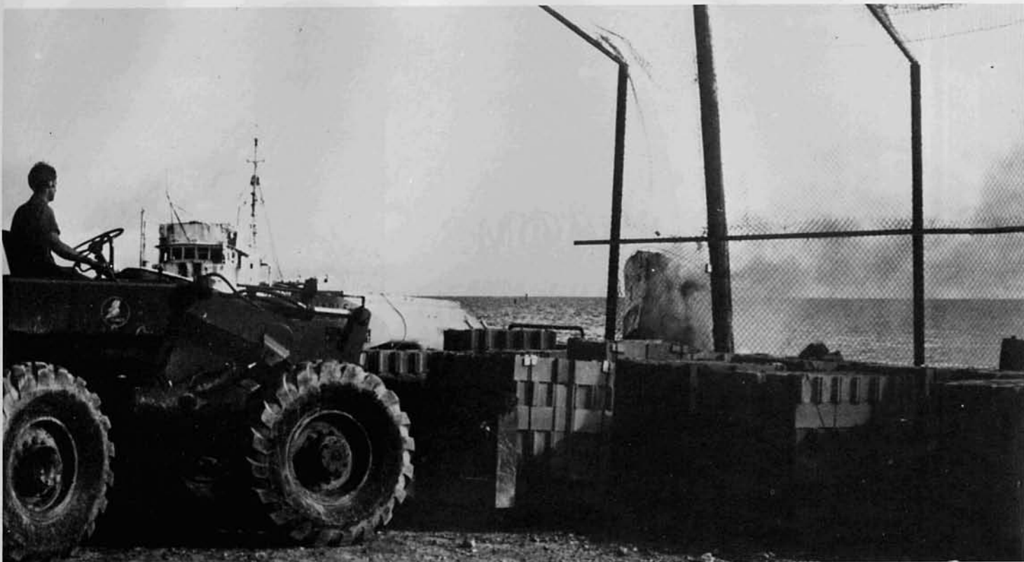
Staging concrete blocks for construction projects in the out-islands
