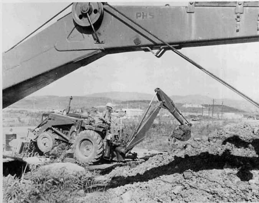
Ditch-digging for the Fleet Rec Center
