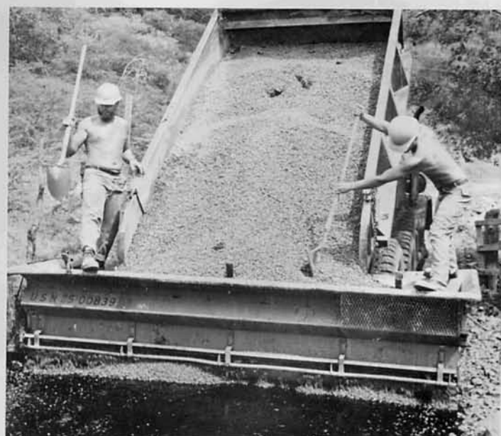
Paving operation
