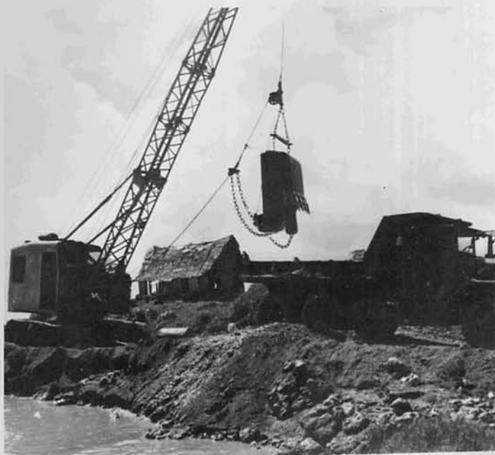
Dredging coral for road surfacing
