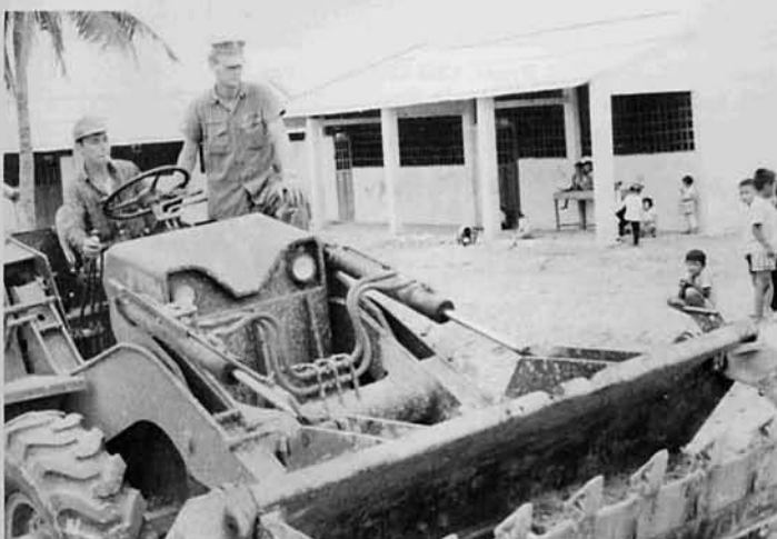
Leveling the school yard at Lagi
