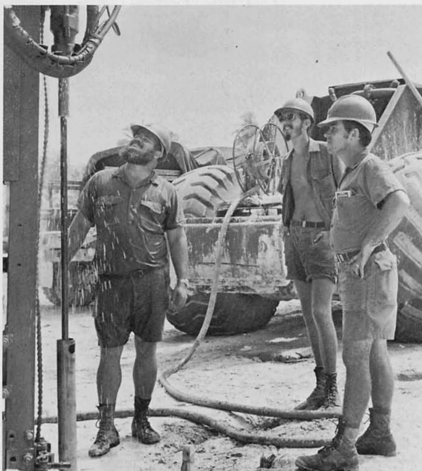
Ivey, Grajewski and Duke drill holes for dynamite charges at the wet well
