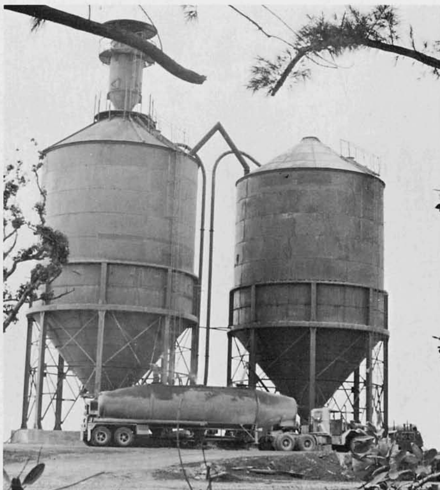
Cement silos — 58,000 cubic feet of storage space
