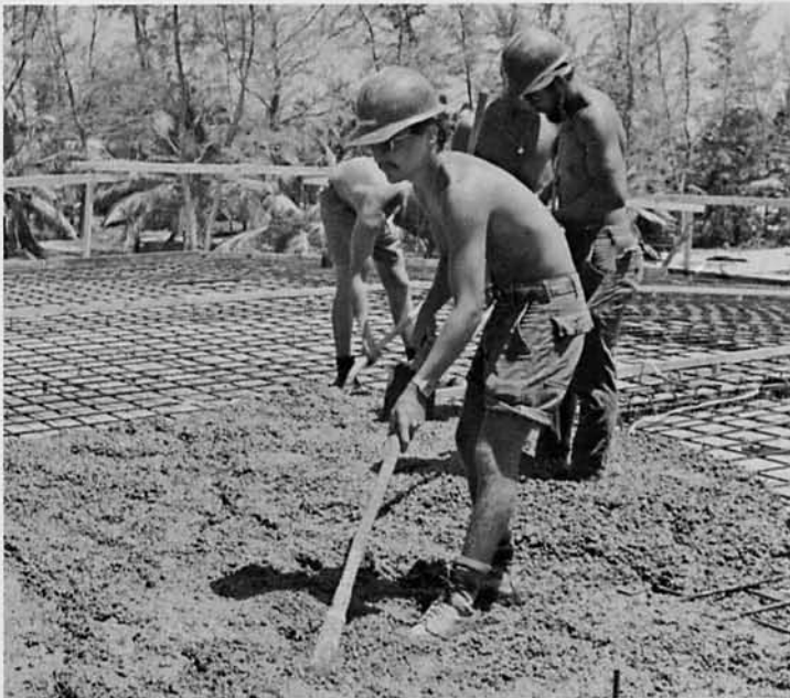
Placing concrete at BEQ #1
