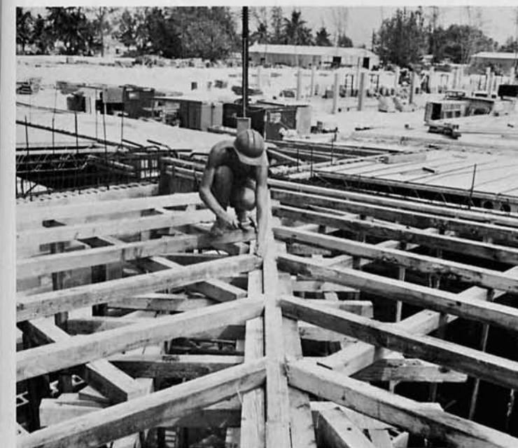
Building forms for a Concrete Roof Pour
