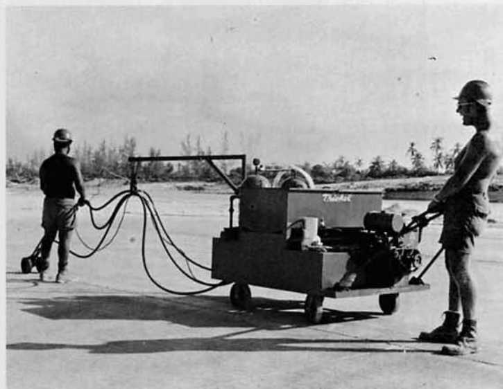
Sealing Joints on the Runway
