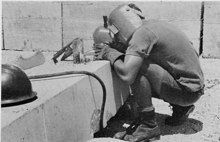
A steelworker welds a lifting eye on a power pole in the C Co. yard.
