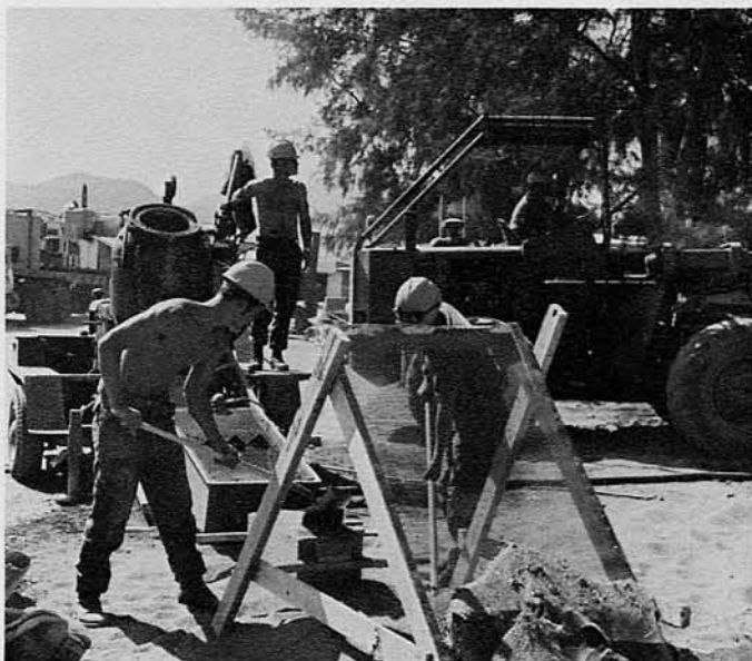
BU1 Viehmann, BUCN Langly and CECN Kirkman preparing to load the skip on the gunnite machine.
