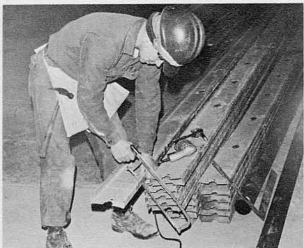
BUCN Moran cutting steel studs.
