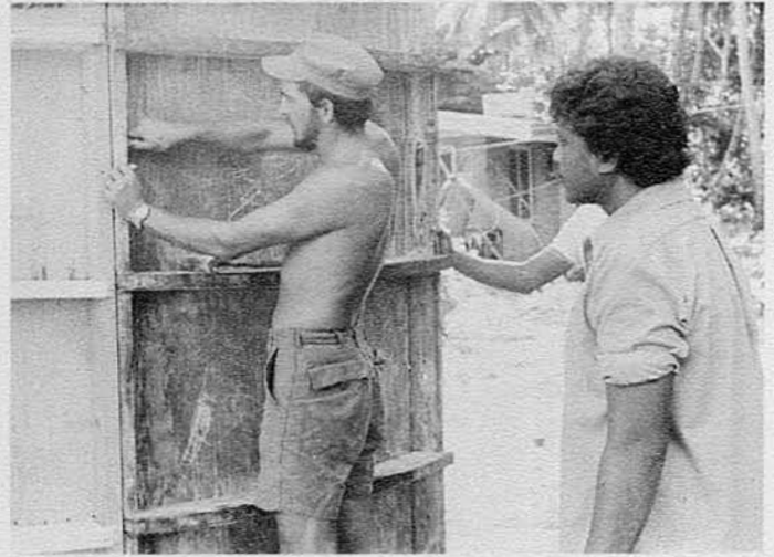
Marlow Draper and trainees bolt together forms for the Udot water tank.
