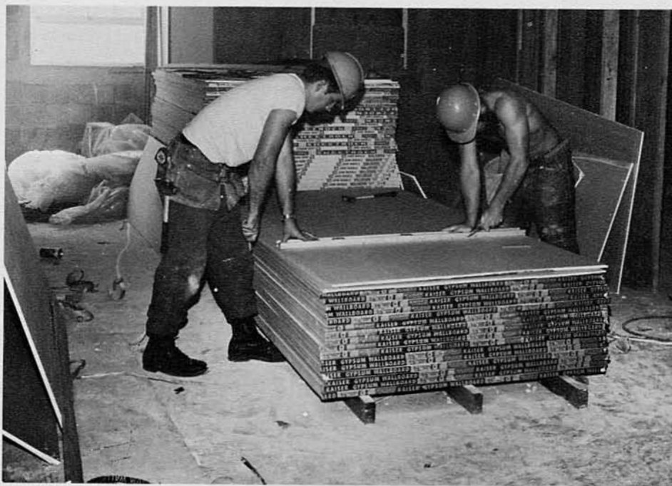
BU3 Stephenson and BUCN Michaud installing sheetrock on second deck.
