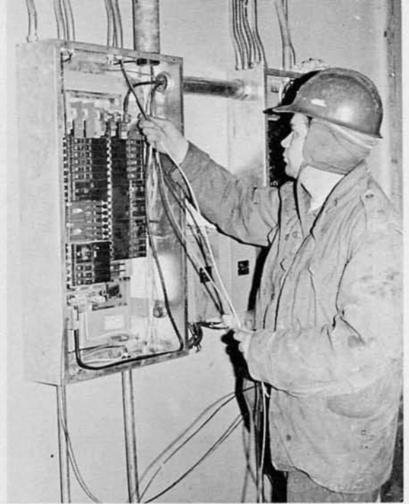
CE3 Dyer pulling wire into electric panel.
