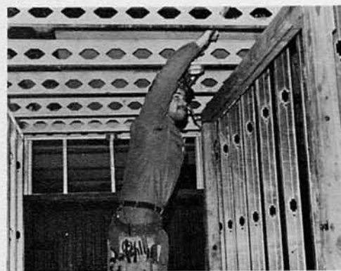
CE3 Drake installing conduit for overhead lighting.
