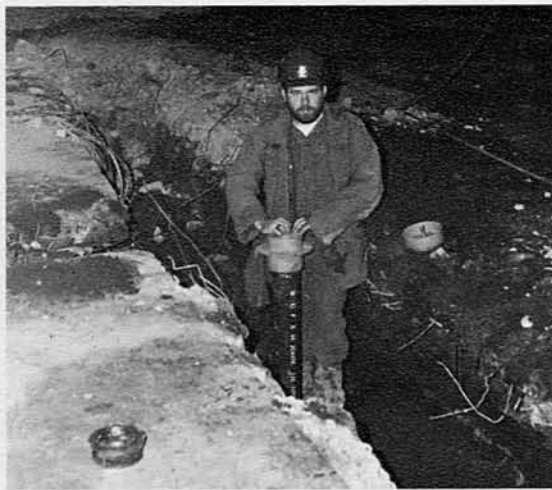
UT2 Bost installing underslab utilities.
