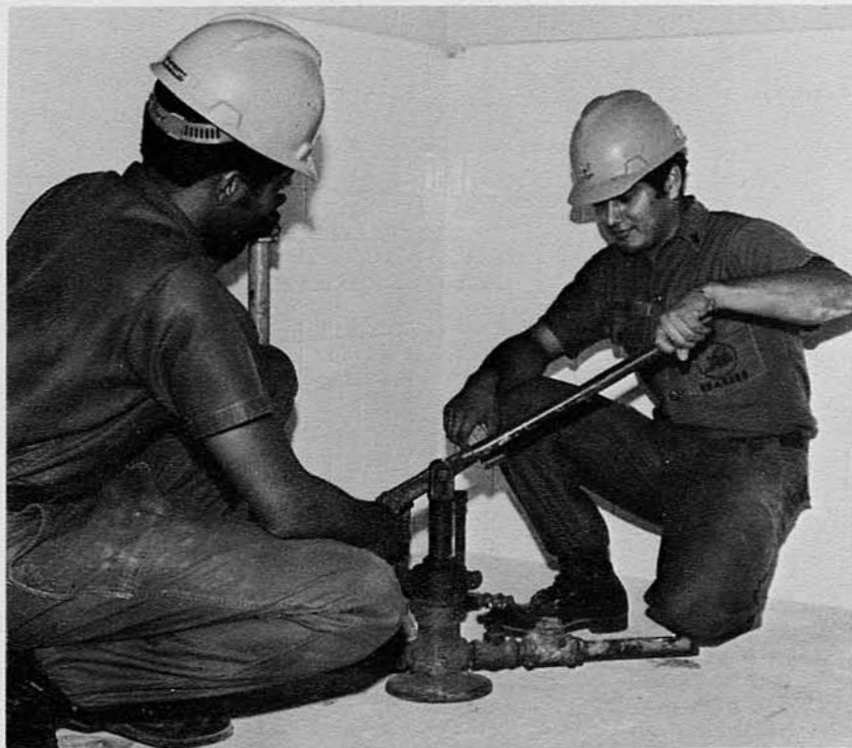
UT3 Telles and UTCN Willett preparing for hydrostatic test of water piping system.
