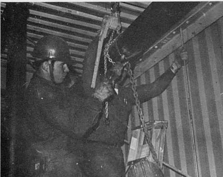
UT2 Fountain and UT2 Lewis installing trunk line on fire protection system.
