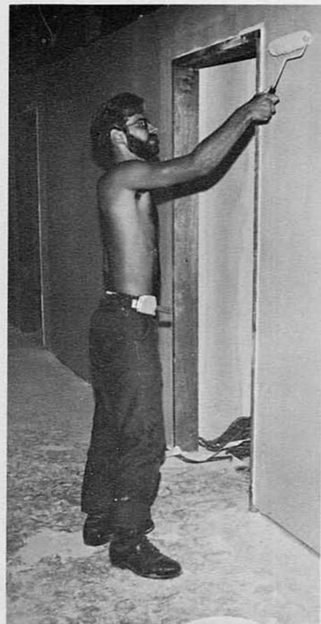
BU3 Wyborski priming sheetrock in preparation for painting.
