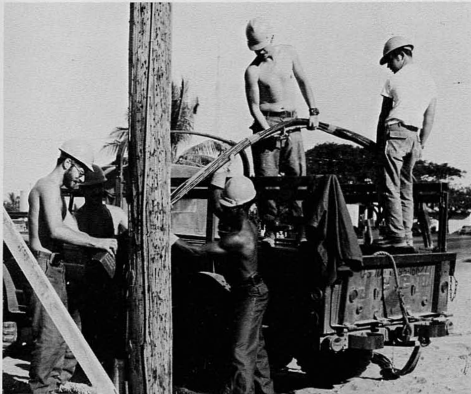
CECN Kirkman checking the permanent power tie-in.
