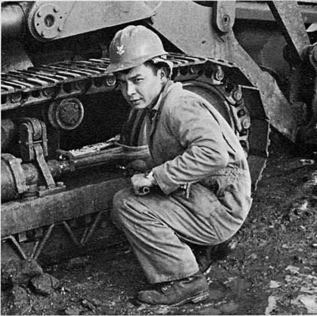
CM2 Edmundo Pingul greasing Case loader.
