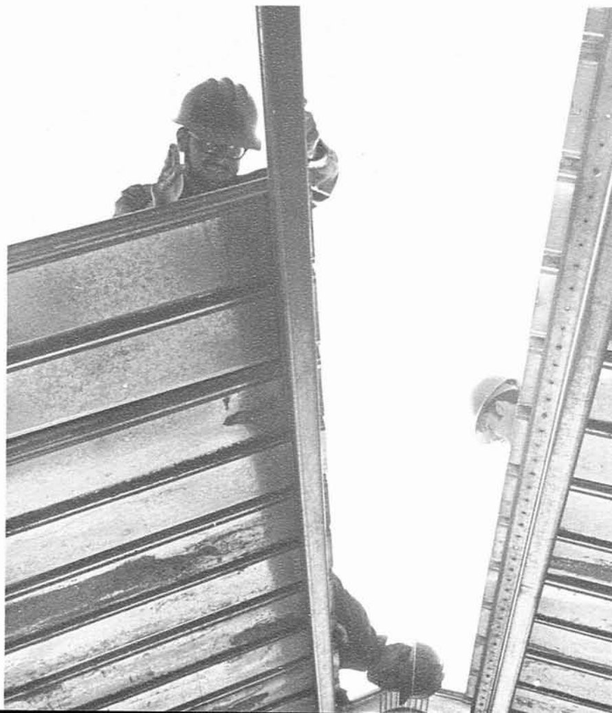
The new Collateral Equipage Building taking shape
