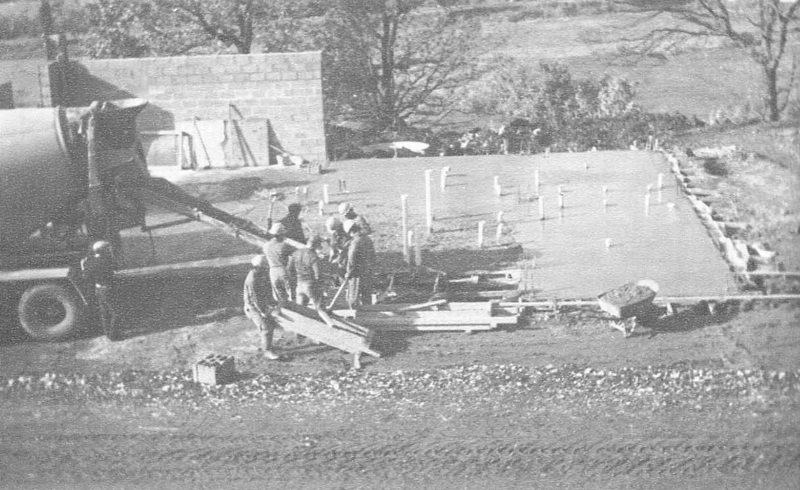
Being poured is the slab for the MULTI-PURPOSE BUILDING project at Gaeta
