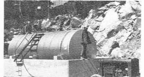
Tank in place
