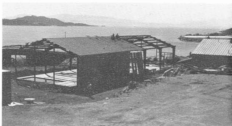
Sheeting the walls and roof
