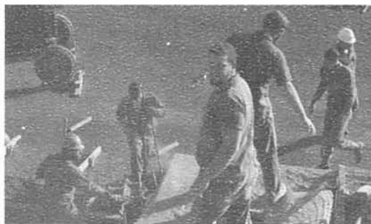
Raymo loading cement
