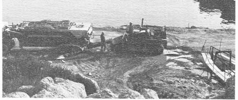
Loading the front-end loader
