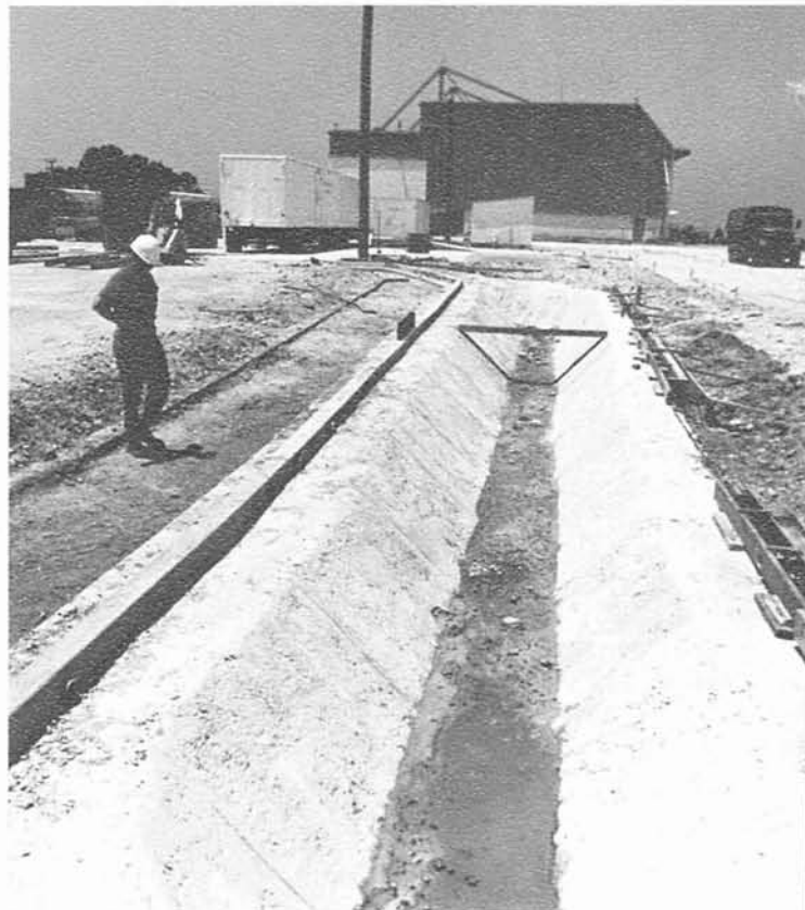
Curbing and form work at the MMF site
