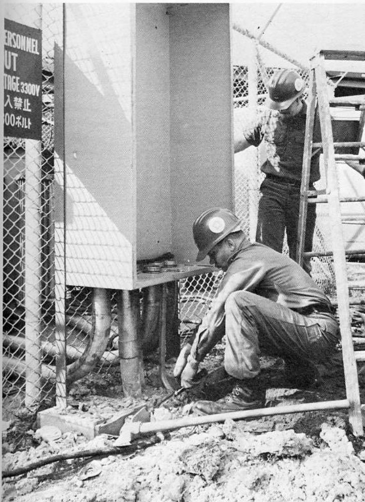
Conduit for the Generator Slabs.
