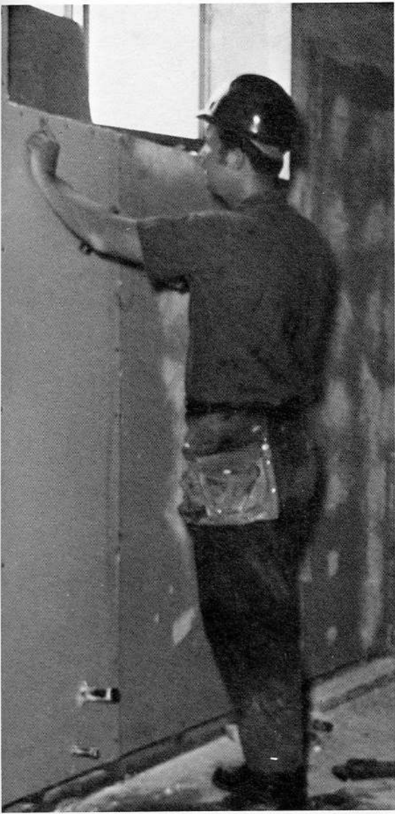
Nailing up sheetrock walls.
