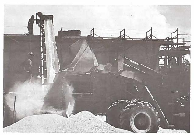
Front-end loader and conveyor belt supply gravel for a built-up roof placement at the EM Club.
