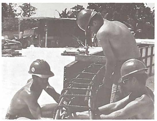
Three Delta men secure rebar that will add strength to the foundation ring at POL. Three rings are completed five more remain to be placed.
