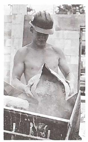
BUCN Brian Spence mixes mortar for block laying at the final water treatment plant.
