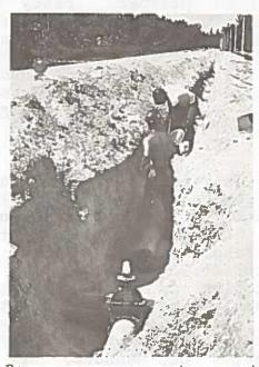
Men of Bravo company put many hours into this project - - the water line for the new laundry stretching about three miles from the canton-ment area. It was completed May 1.
