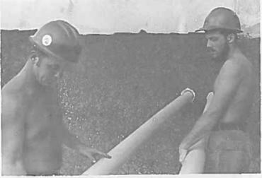
CE2 William Burke and CE3 Tom Goodwin install PVC conduit into the pool's mechanical room.
