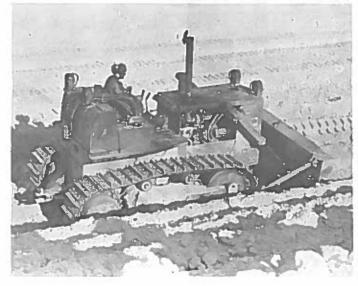
Equipment operator runs an HD-21 bulldozer at the Point Marianne dredge pile. Alfa company is supporting the POL project by hauling over 200,000 cubic yards of coral fill.
