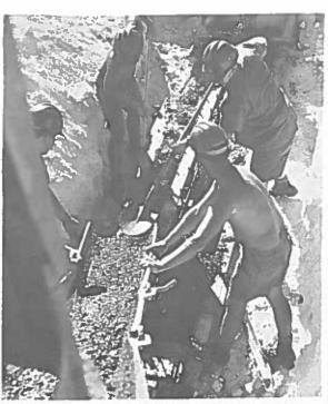
Concrete flows from a transit mixer and is placed by men of Charlie company during BEQ construction.
