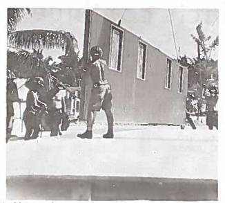
Wall section of a portahut is installed by Charlie company men in the camp area, with support from an Alfa company crane.
