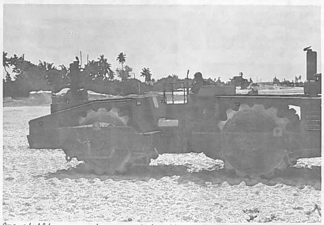
One of Alfa company's segmented rollers toils across the POL project area. Coral fill is compacted to bring the site up to grade. Civilian contractors will begin the steel tank construction of eight, 80,000 barrel-capacity fuel tanks about Sept. 1.
