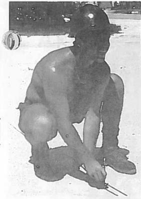
Stretching the tape to its limit, FACN Jerry Wolfe marks the point where the corner of a structure ill be placed.
