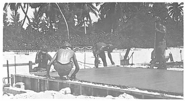
Charlie company's BEO crew finishes the surface of a barracks deck slab.
