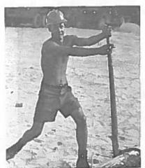
CECR Rick Miller uses a canthook to hold a lightpole in position while it is prepared for erection.
