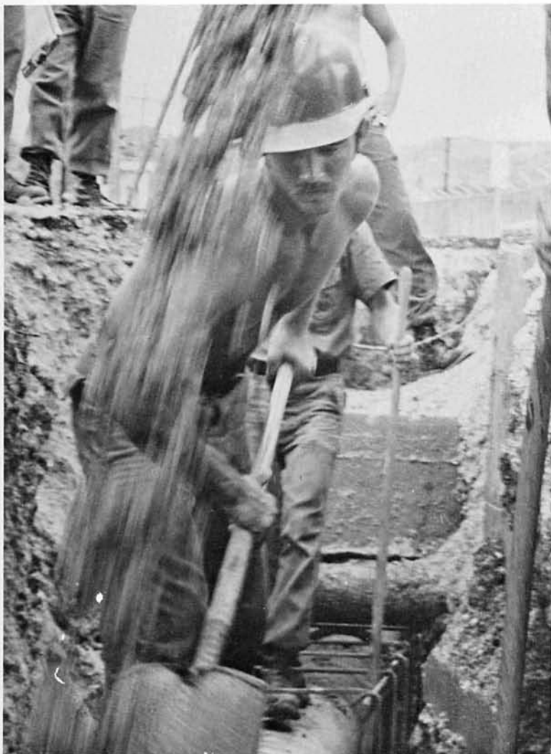
Left: As concrete rains from the chute, UTCN Whitehouse spreads it over pipe with a shovel.
