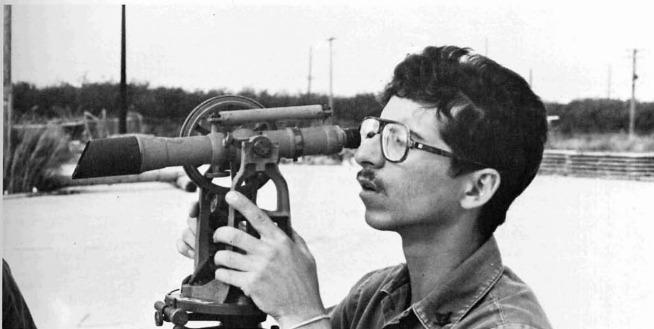
EA3 Rusnak adjusts his transit while taking readings at the warehouse for the engineering department.
