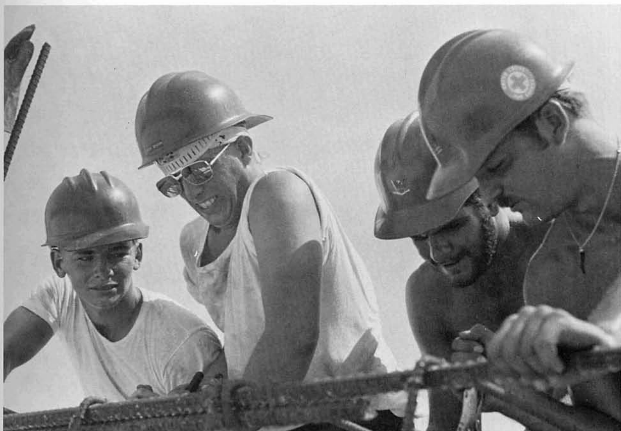
A tedious but necessary task: tying together reinforcing steel before placement of concrete. Working on the job are BUCN Wilhelm, BUCN Brown, BU3 Dellapiazza and BU2 Bouley.
