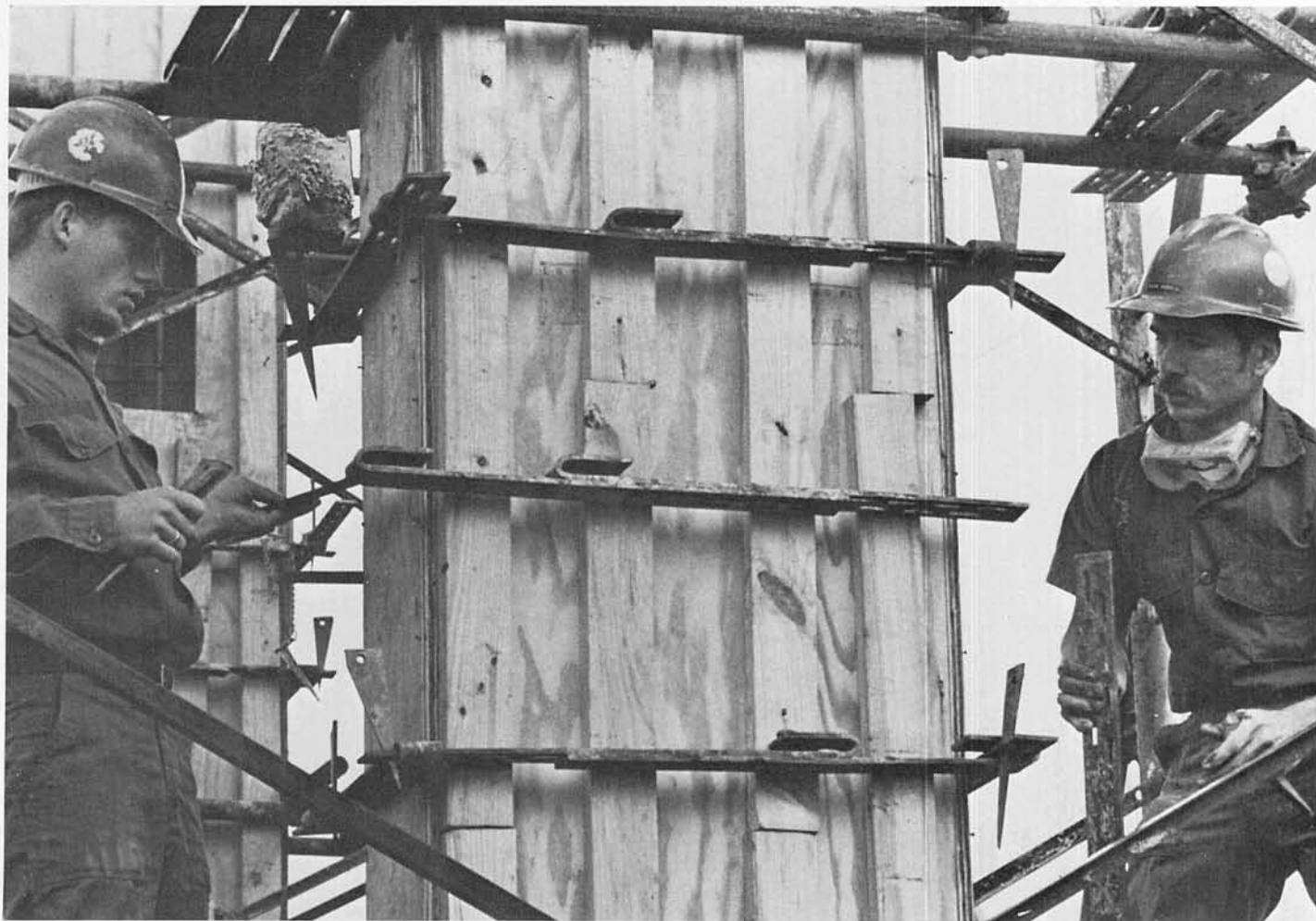
BUCN Ed Spurlock and BU3 John Kochis getting ready to pour columns at the fire shed project.
