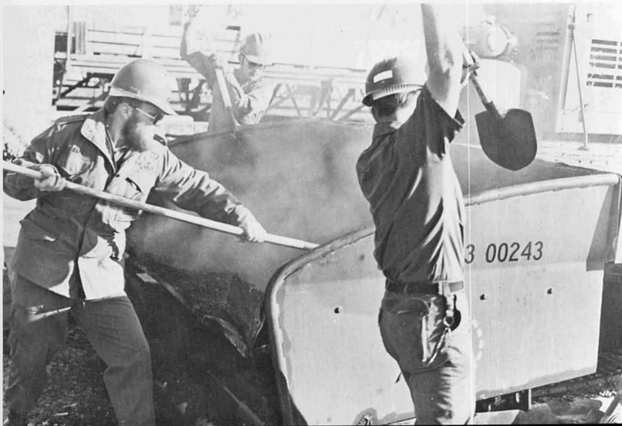
Emptying the hopper before the next asphalt truck arrives; E0CA Souza, E0CN Barrows, E0CN Oris and E03 Hall.
