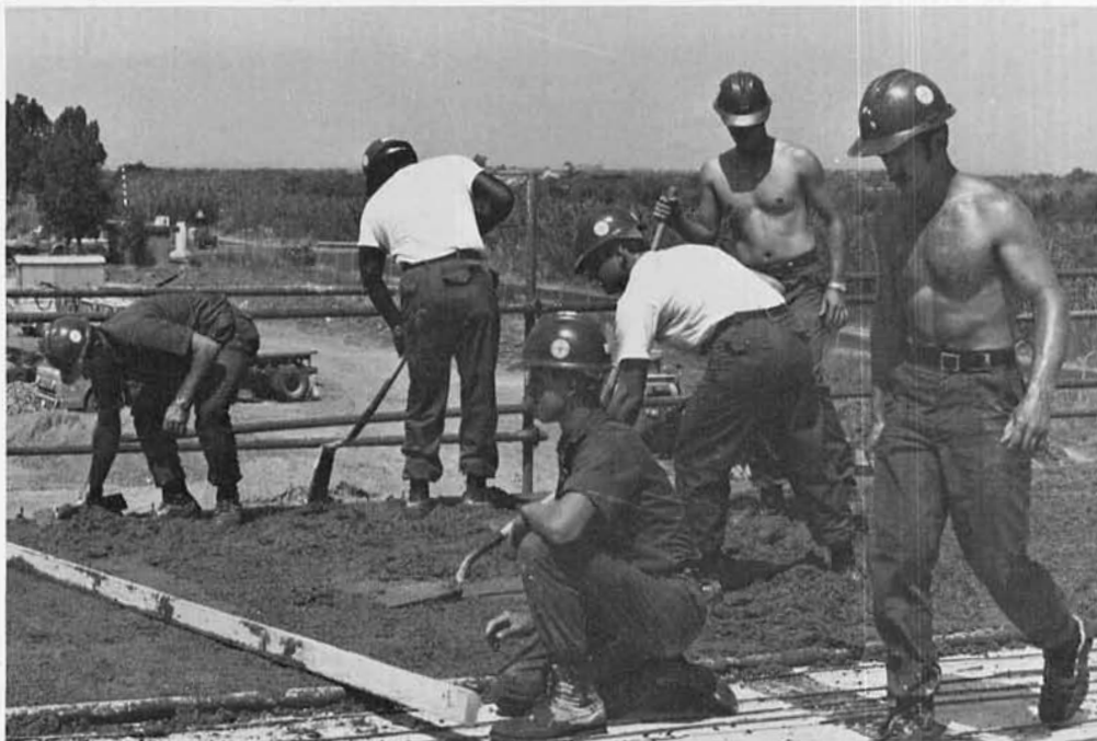
BU1 McBride, BU2 Hill, BUCN Redding, BU3 Lollar, SW2 Paris, and BU3 Kochis placing concrete cap on the refueler shop roof.
