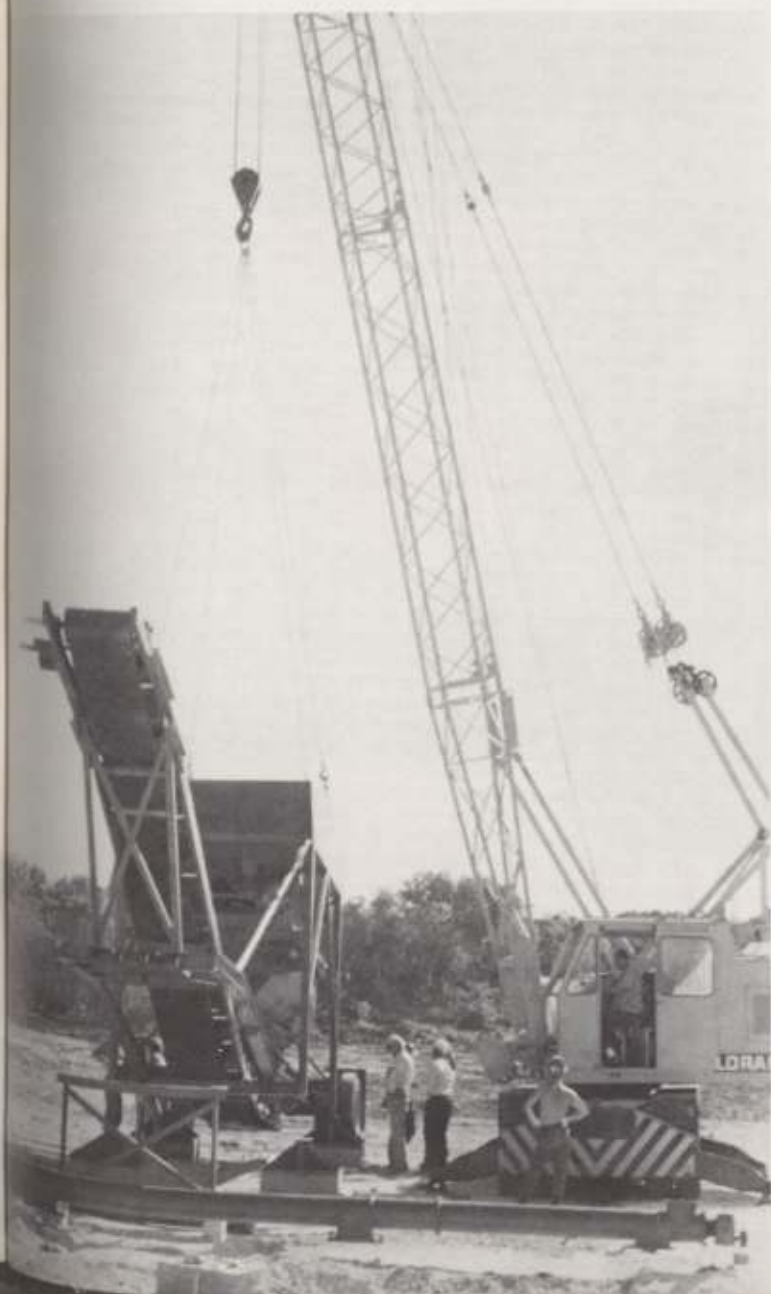
Setting the aggregate batch plant on footers.
