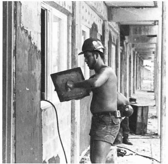
BU2 Edward Spurlock plastering masonry walls.
