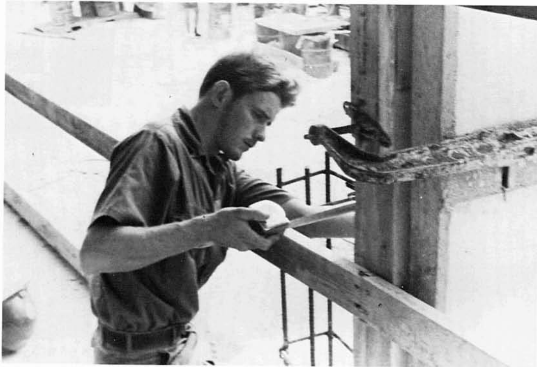
BU3 Mann measures for the concrete handrails to be placed.
