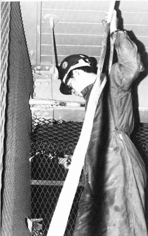
SW2 Jeff Perkins strips the sea plane hangar of expanded metal for reuse elsewhere.
