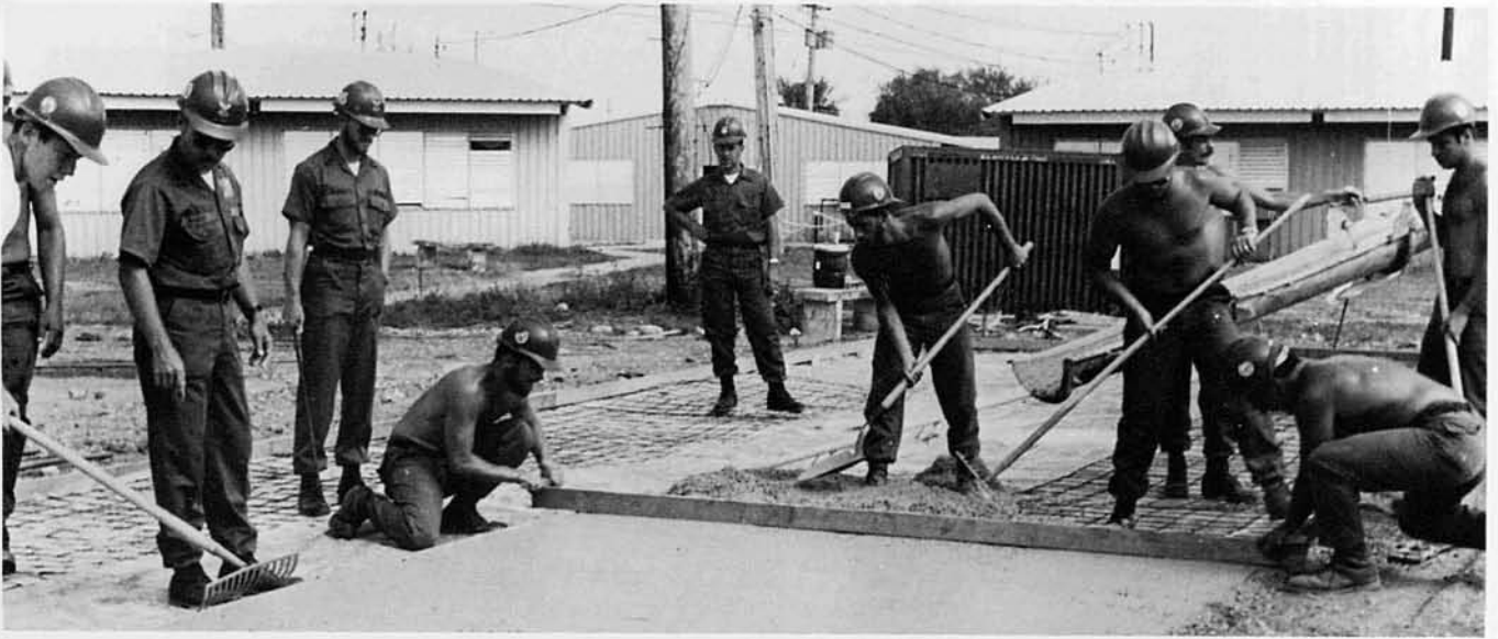
Charlie Company crew members smooth out a concrete pour under the watchful eyes of Quality Control.
