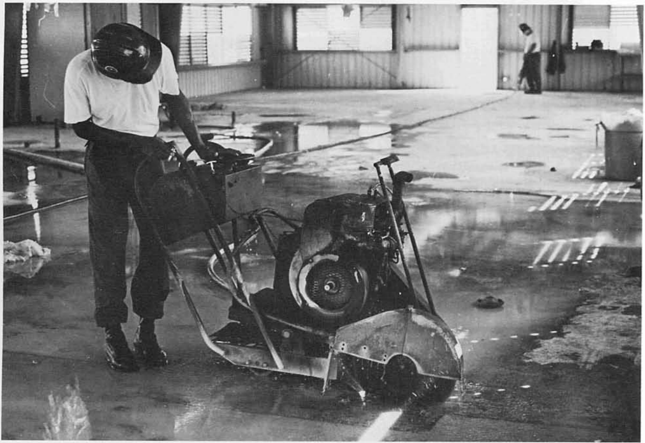
The concrete slab is cut in the Barracks 519 rehab project.
