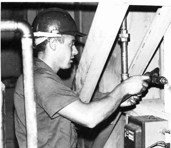
UT3 Danny Thompson makes a connection to the Tire Shop's air compressor.
