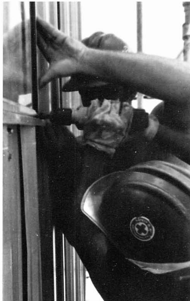
Two steelworkers install window in PEB.
