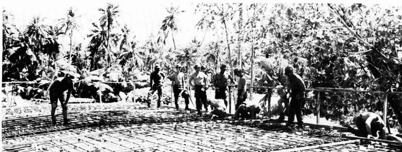
The crew readies the roof for "the pour".
