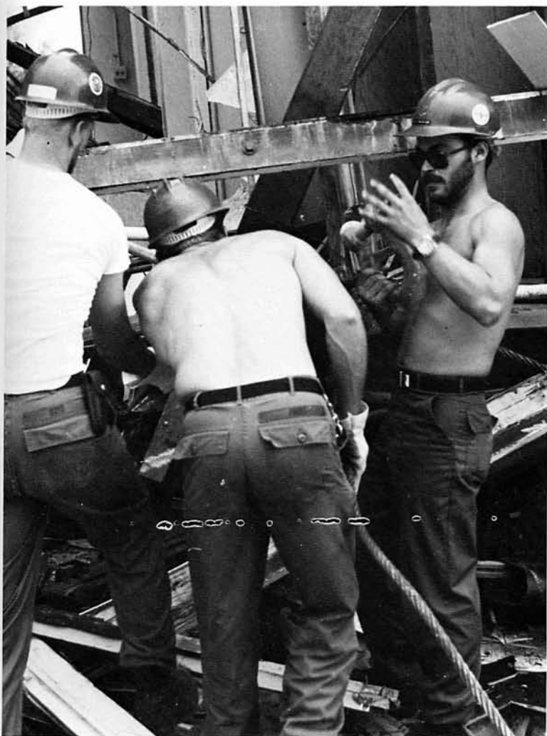
EO3 Palaniuk connects the cable from the dozer at the BOQ demolition site.
