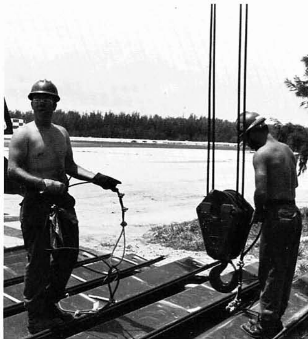
BUCN Scott Hughes and EO3 J. D. Palaniuk prime the sheetpile for installation.
