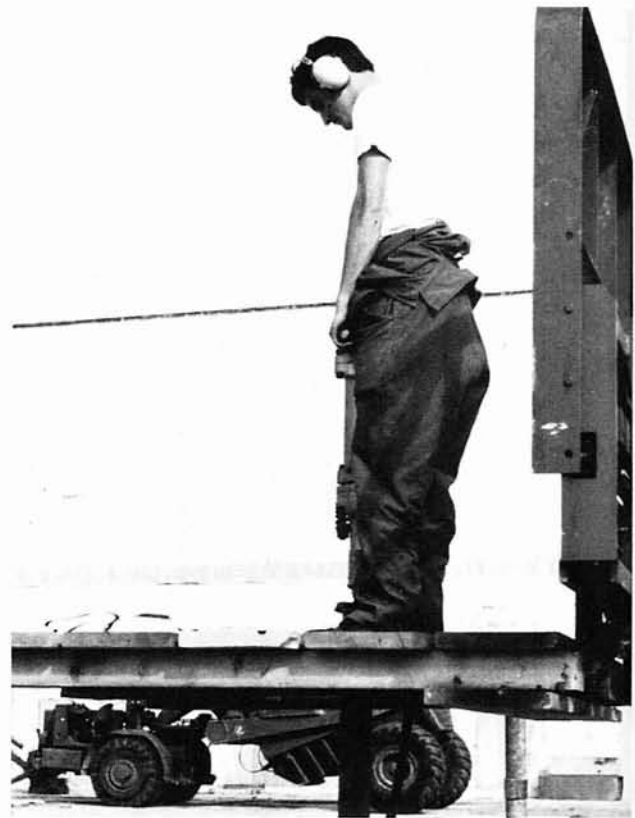
SWCN Mike Aukema lines up and levels a fence post to be driven.
