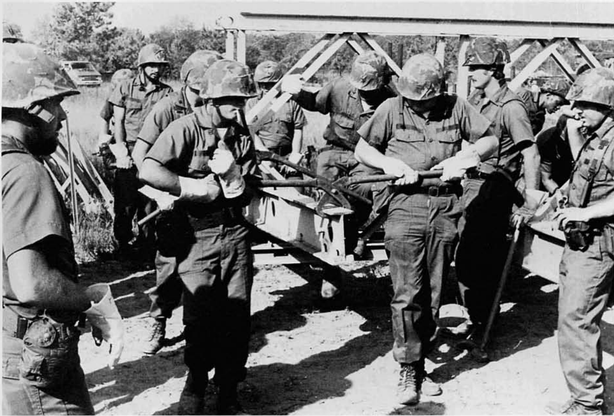
NMCB-62 Seabees construct a Bailey bridge during contingency construction training in homeport.
