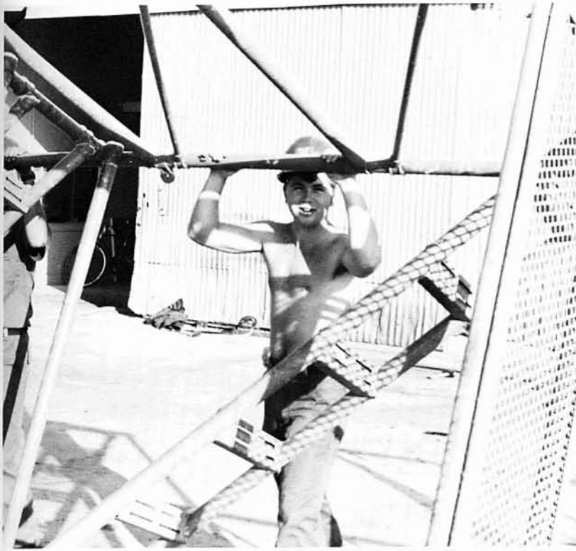
BU3 John Coutts assembles the scaffolding for the hangar painting job.
