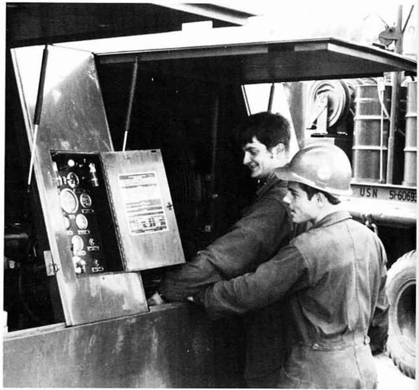
CMCN Kevin Baker and CMCN Dennis Doyle prepare the piledriver's air compressor for use.
