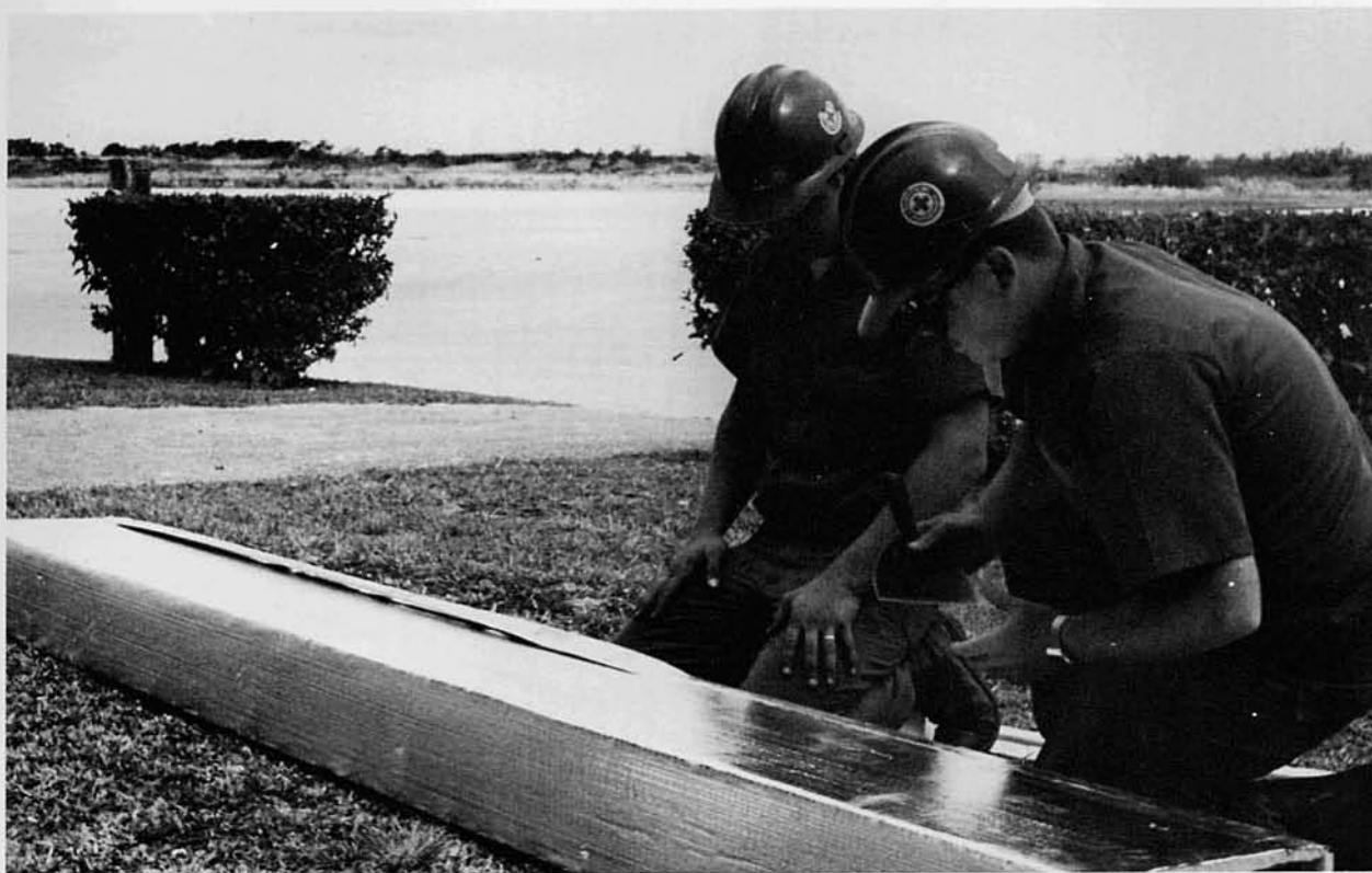
UTCN David Johnson (left) and UT3 Dickson put the finishing touches on a fiber duct.
