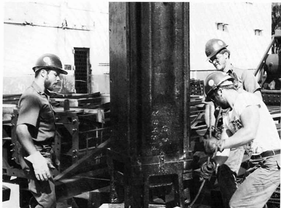
EO3 Tom Weber, EO3 Terry Green and EO3 Tom Trayer assemble the pile-driving hammer for the long job ahead.
