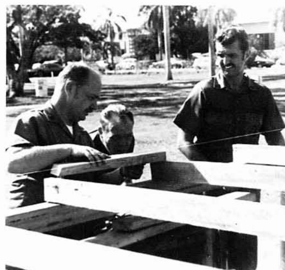
BU1 Mike Manley, EO1 Bob Williams and CEC Lloyd Bigford check out the plumb line for the stage foundation for the Festival of the Arts.
