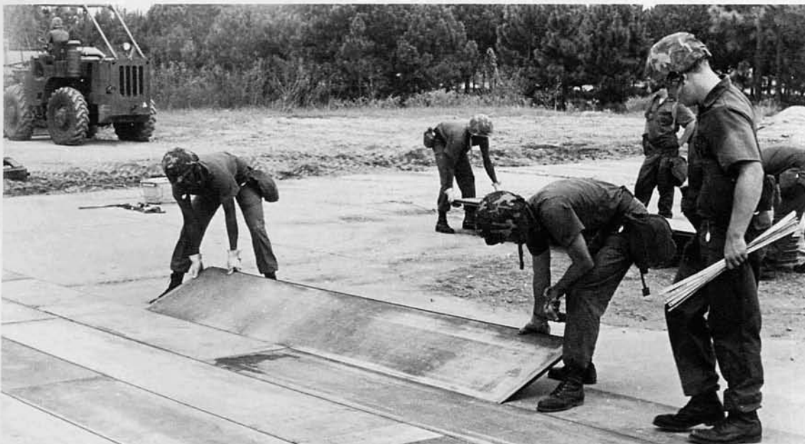
Rapid runway repair team members place a mat into position.
