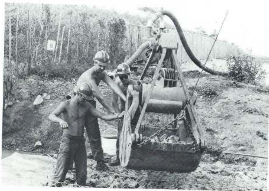
Charlie Company crew members fill up gabions with rocks at the Security Fence Line project.
