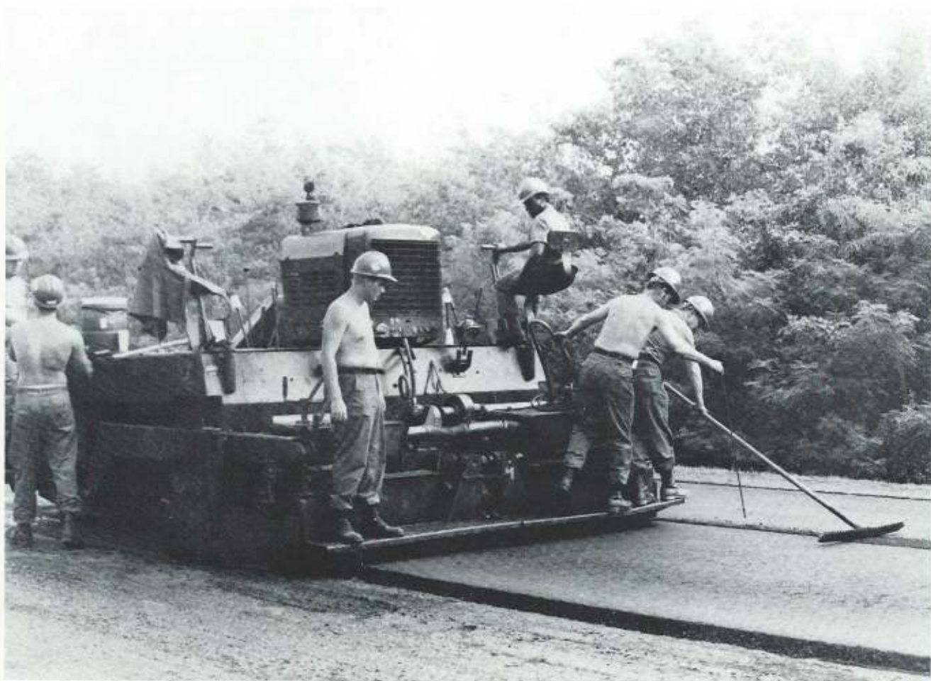
CM2 Harold Brown (left) and CMCN David Reavis pull an engine on a scraper (above). The Alfa Company Tow Way Road crew lays down asphalt (below).
