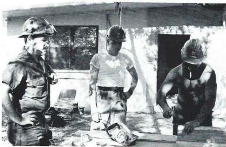
Base Housing project crew members assemble forms.
