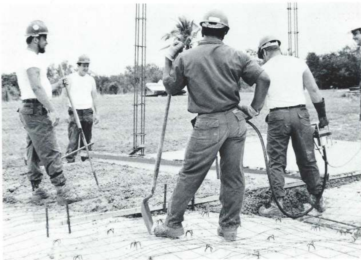
Det Andros crew members construct a CMU block storage building at Site 2.
