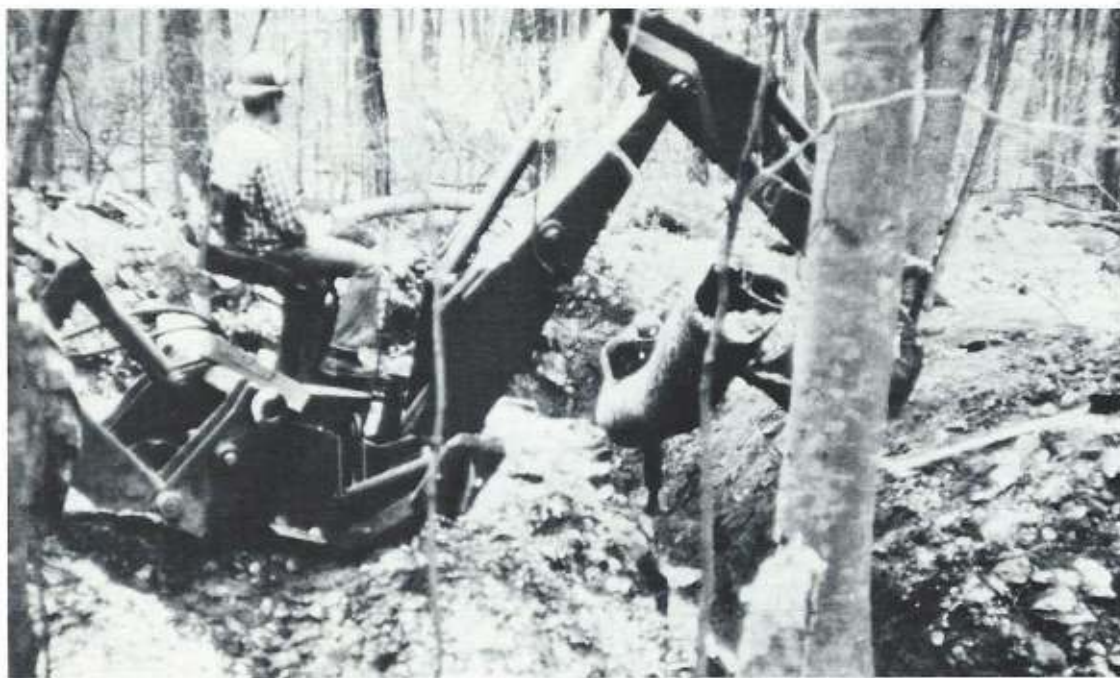
DET Thurmont Minutemen repair the roadbed and replace culverts at the National Park Service site.
