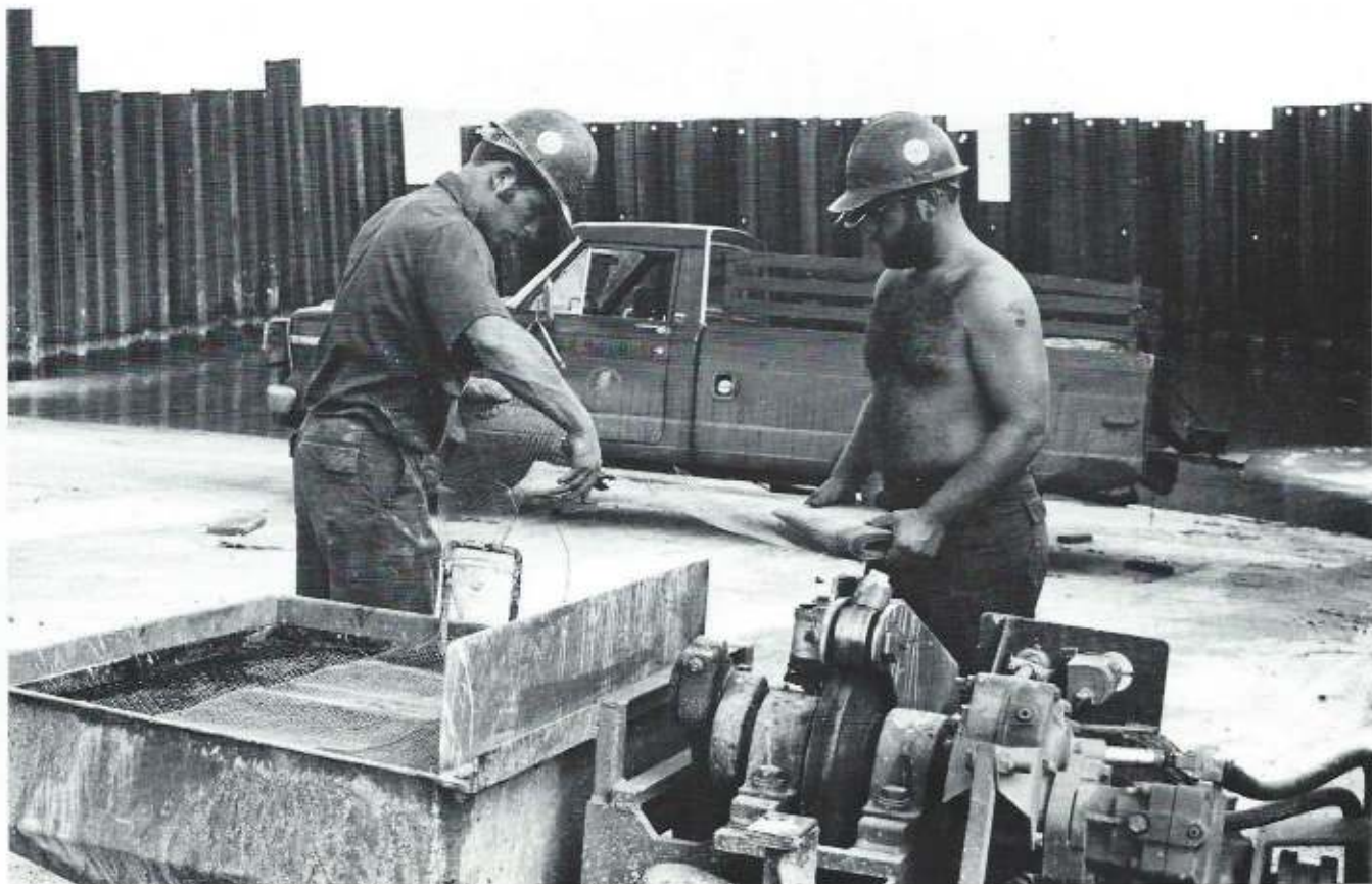
DET Vieques members prepare a grout pump.
