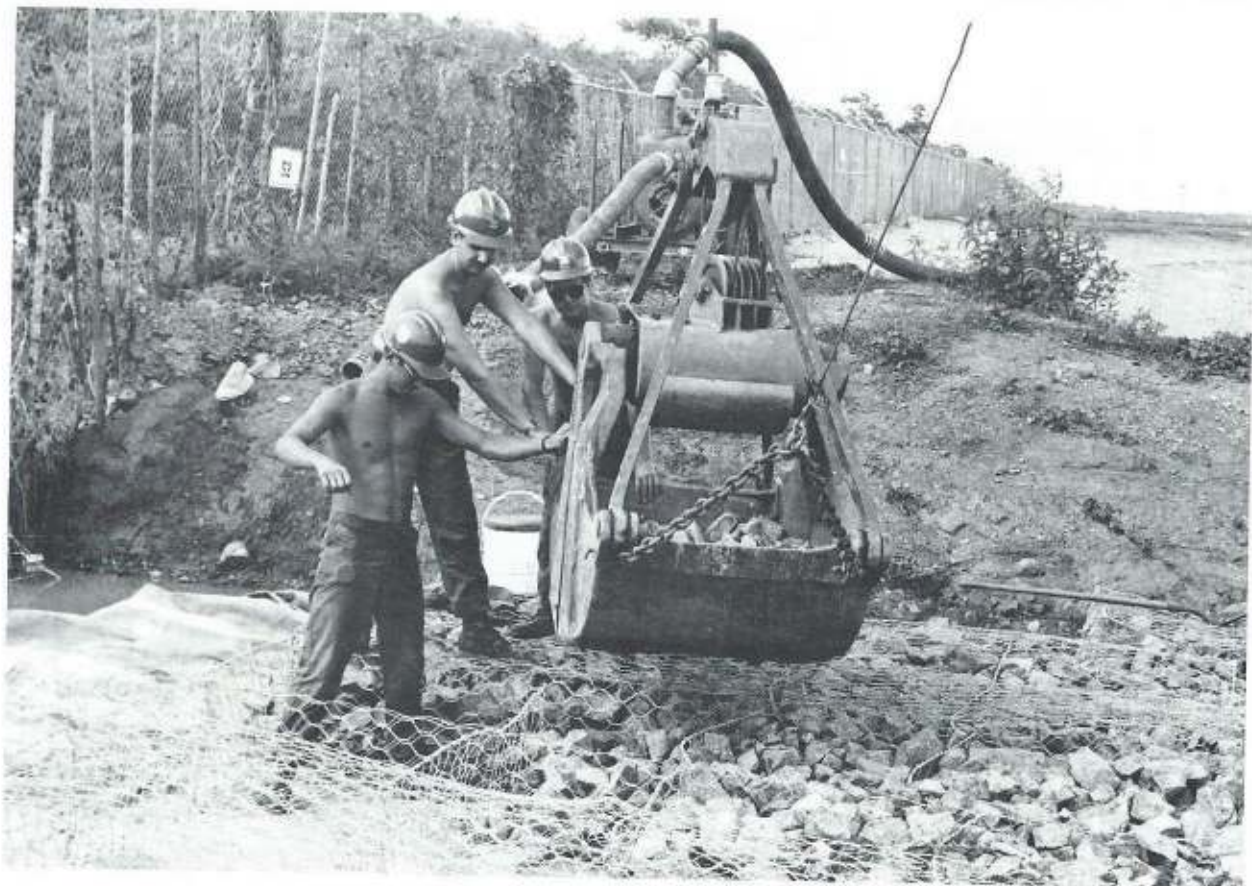
Alfa Company lays down asphalt at the Tow Way Road project (top). A gabion crew fills a gabion with rock at the Security Fence project (above).
