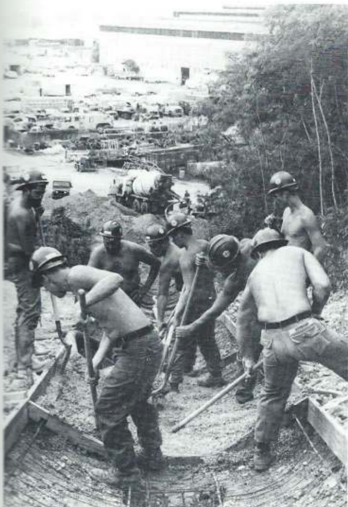
Charlie Company crew members spread concrete at the Industrial Drainage project (left). BU3 Clarence Bouse cleans the mixer after making a batch of mortar (above).
