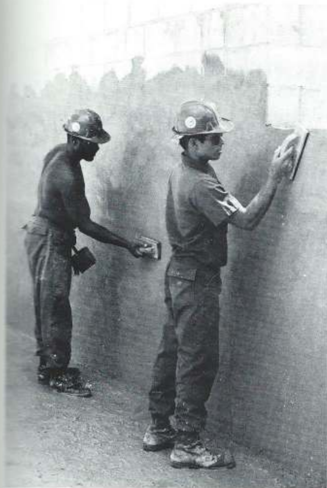
BU2 Nelson Carter (left) and BU3 Ysmael Salas grout to seal block at the Ops Storage building project (above). Charlie Company crew members pour concrete steps at the Seabreeze Addition project (right).
