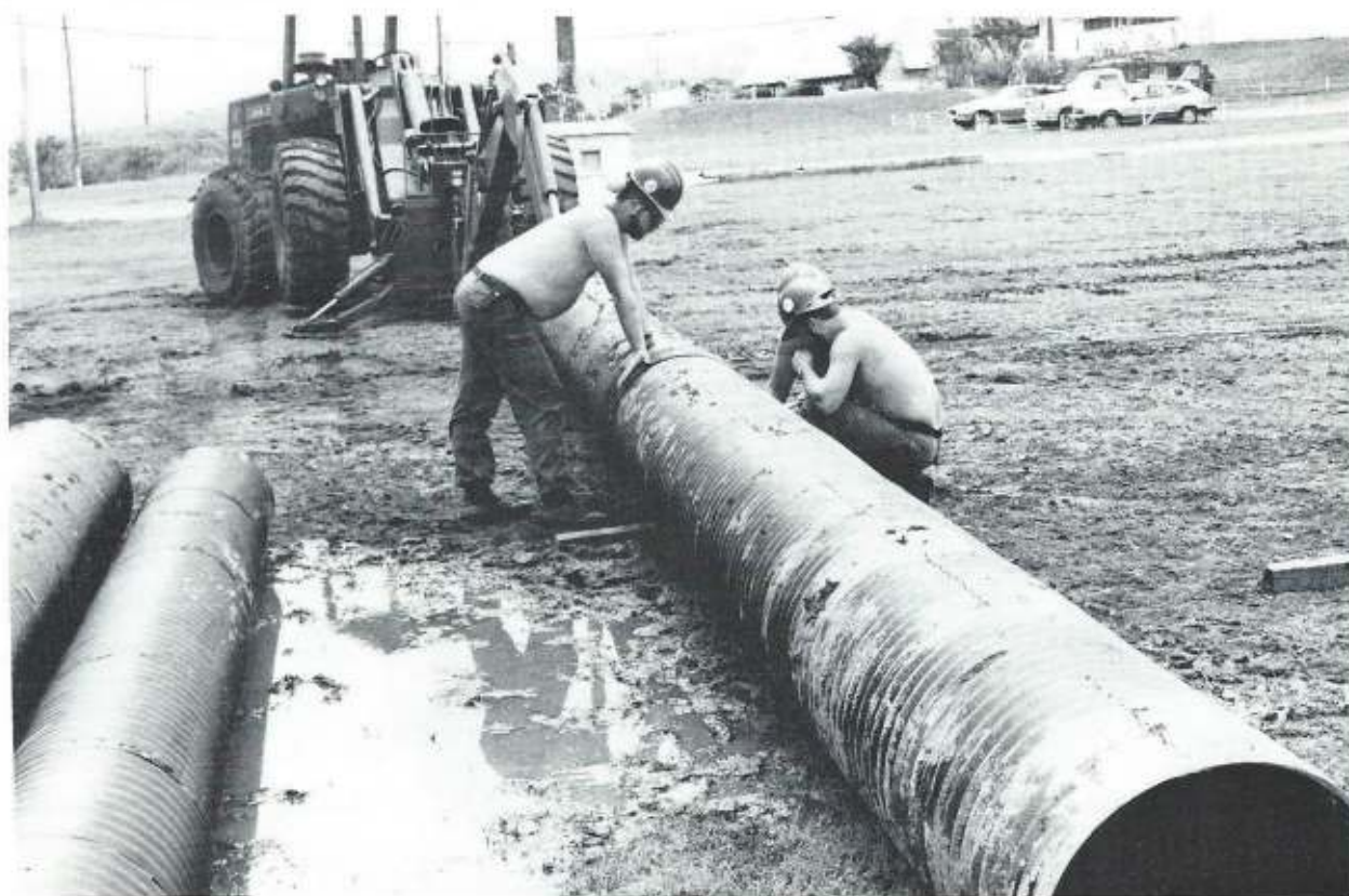
DET Vieques Seabees band together a pipe extension.
