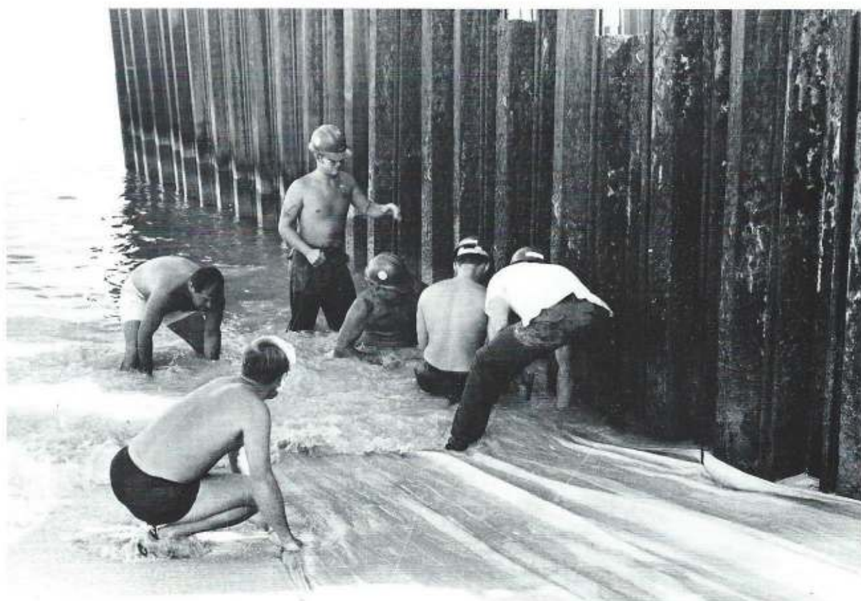
DET Vieques Minutemen lay down fabric at the pier project.
