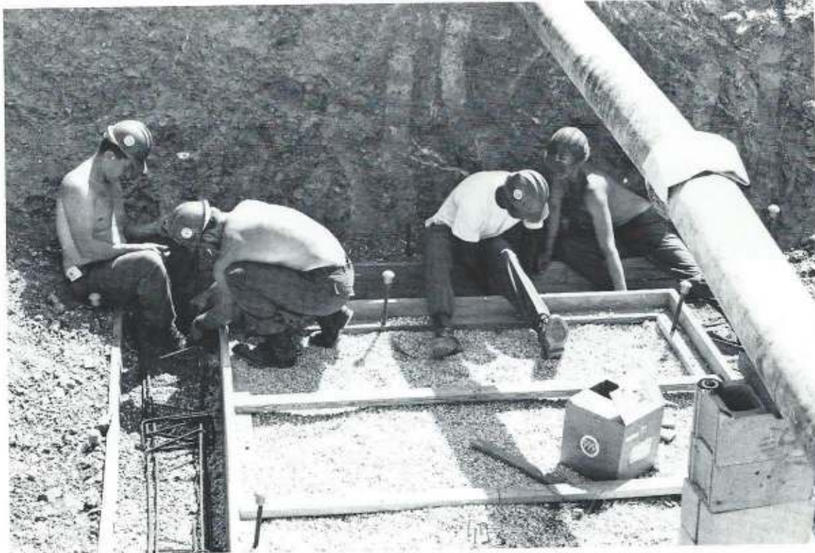
The Water Pit crew constructs forms for the foundation.
