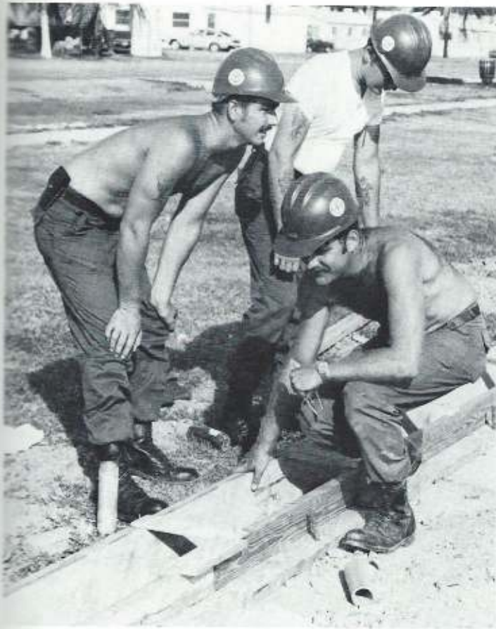
A Bravo Company crew lays forms for a concrete curb at the Enlisted Dining Facility parking lot.
