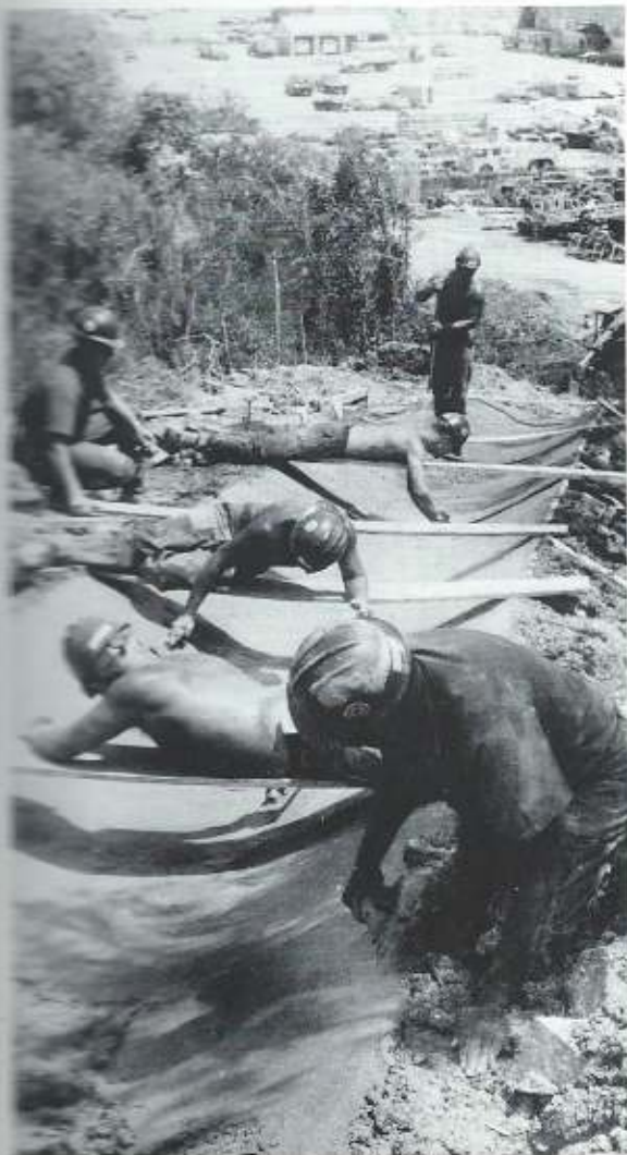
Bravo Company utilitiesmen smooth up concrete on Magic Mountain (left). Equipment operators fill gabions at the Security Fence (above). The gabion crew puts the finishing touches on the special wire construction (below).
