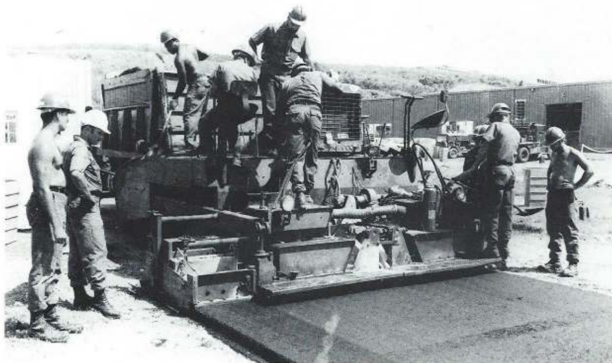
The asphalt crew puts down an overlay at the MWR parking lot.
