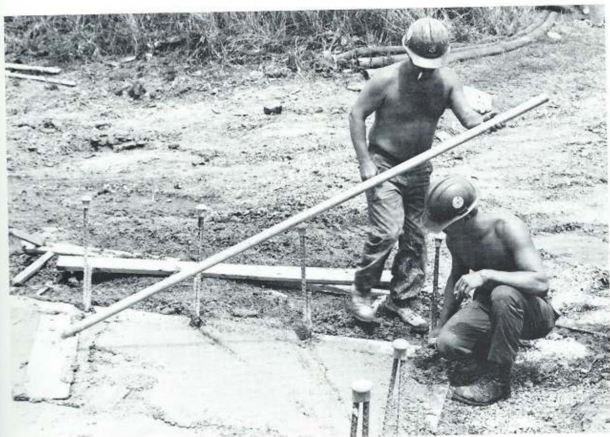
BU2 Terry Jackson sponge floats concrete at the Camp Moscrip Laundry/Linen Bldg. project (above). Charlie Company Minutemen smooth up the foundation at the Dog Kennel (below).
