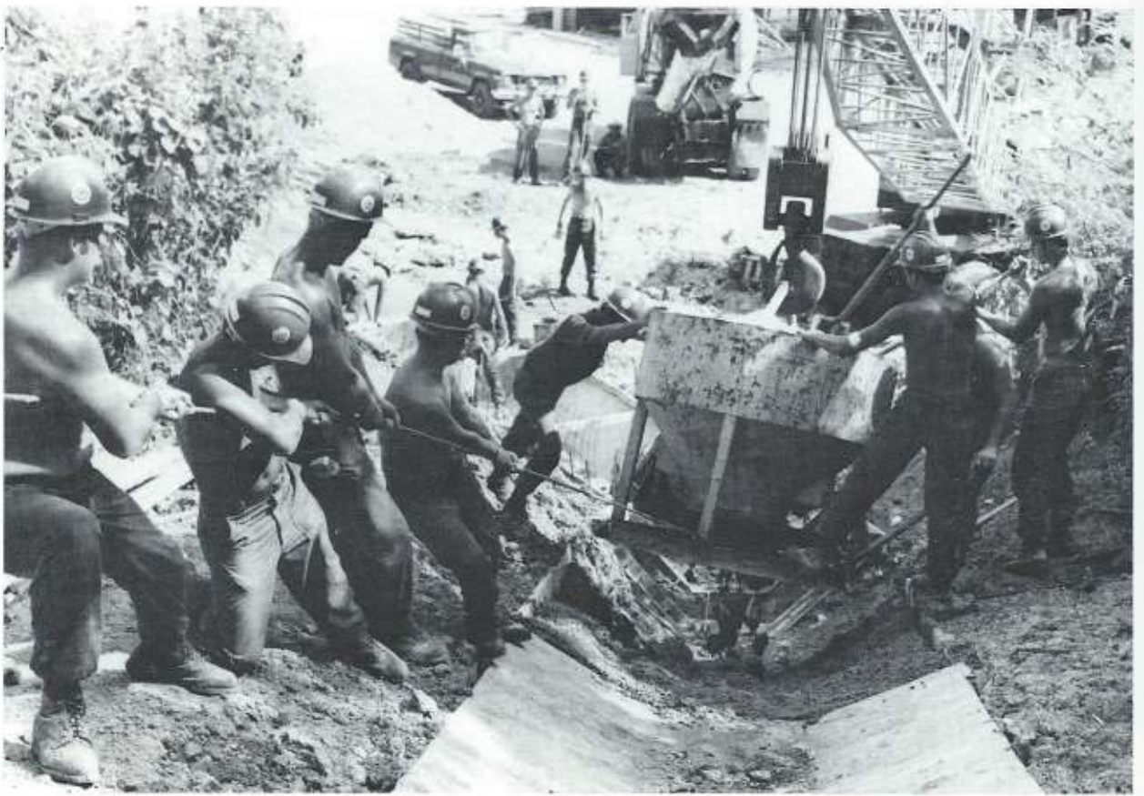
Charlie Company uses a crane and a concrete bucket to place concrete on remote portions of the Industrial Area Drainage project (above). Alfa Company prepares asphalt lay down at the Public Works Department parking lot (below).
