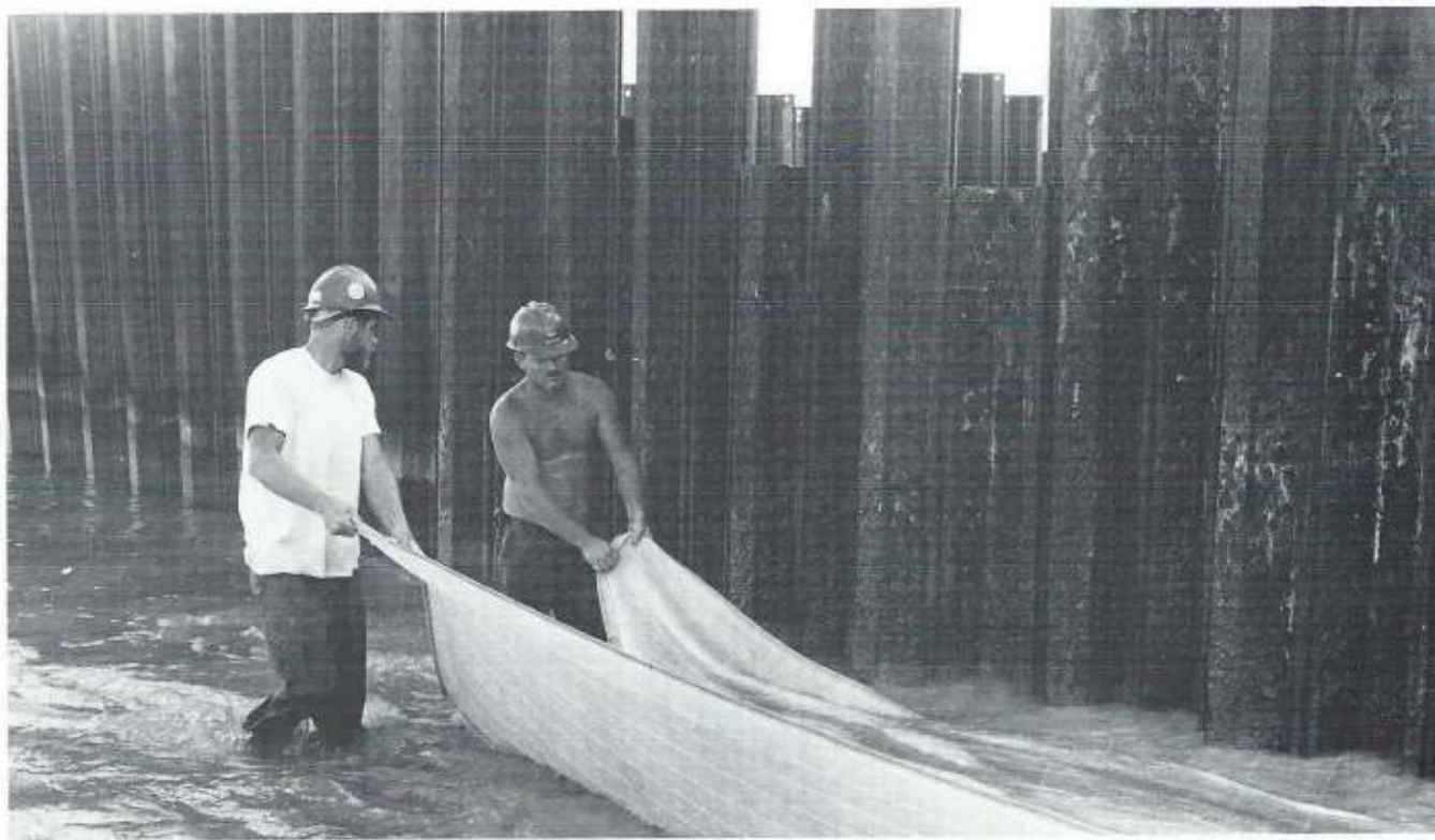
DET Vieques Seabees lay down fabric at the pier.
