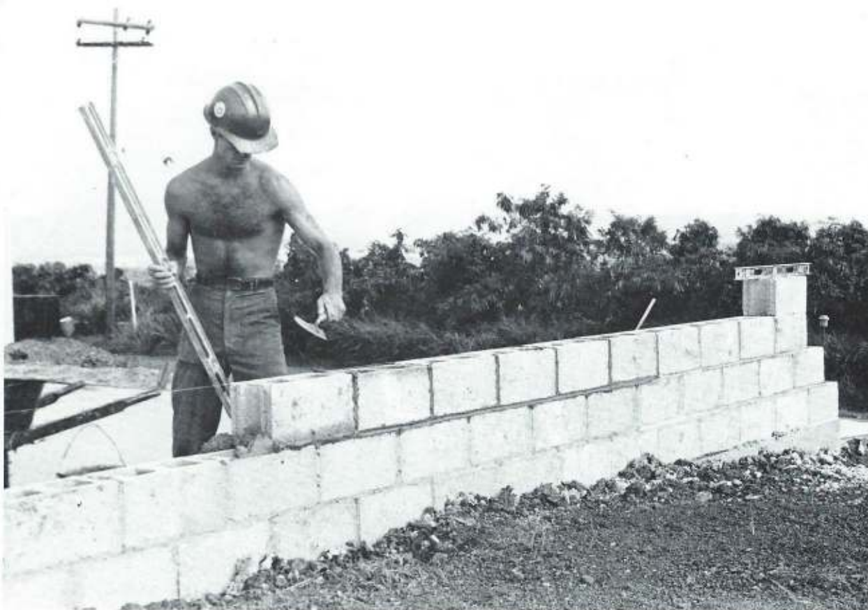
A Charlie Company Minuteman levels concrete blocks at the Seabreeze Club Addition (above). Bravo Company was responsible for Camp Moscrip maintenance such as parking lot improvements (below).
