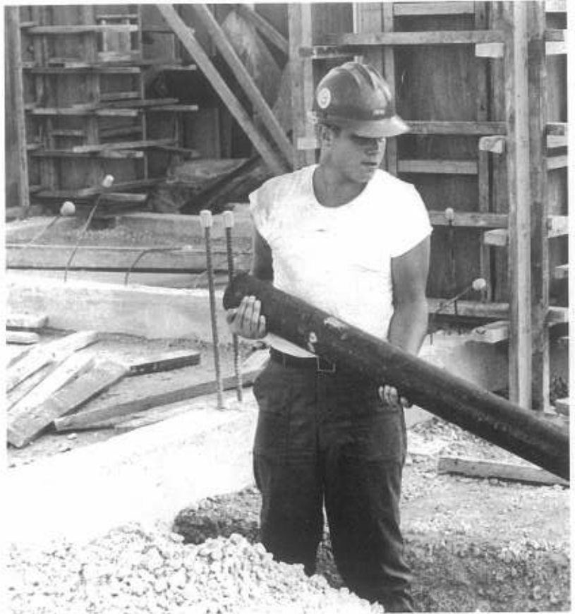
UTCA Beyer places drain pipe prior to slab going in.
