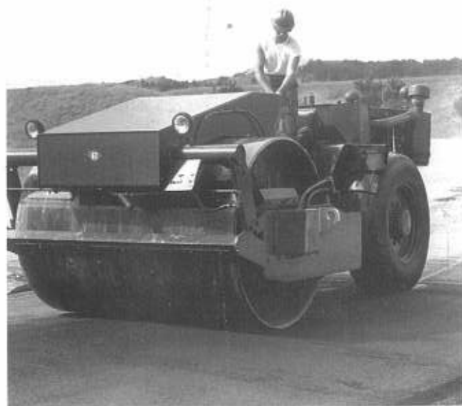
EOCA Rainey makes break down pass on new asphalt.
