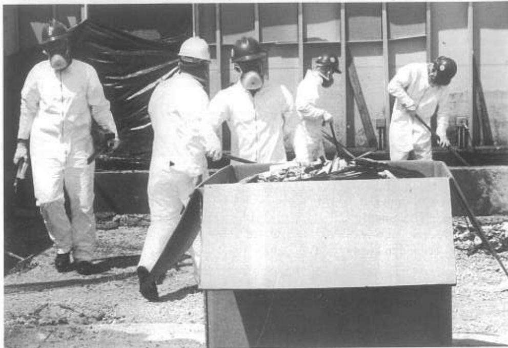
Safety team removes asbestos from T-350 addition project.
