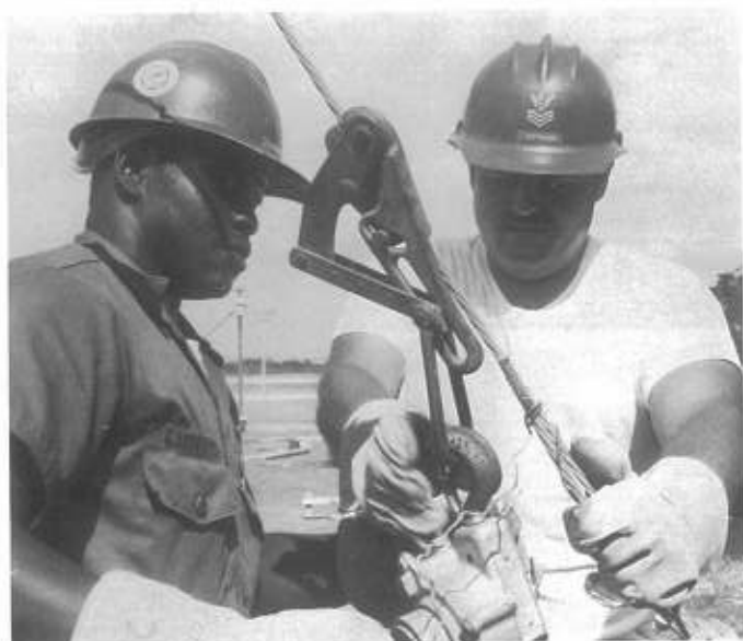
CE1 Patnaude and CECN Carpenter apply tension to guide wire prior to pole removal.
