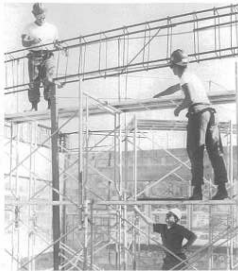
SW3 Campos and SW3 West tie rebar as BUC Kielser Safety Chief looks on.
