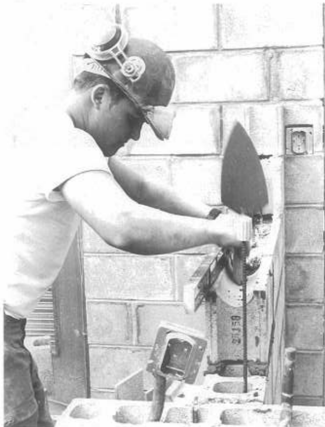
BUCA Wink taps block in level at the pesticide storage project.
