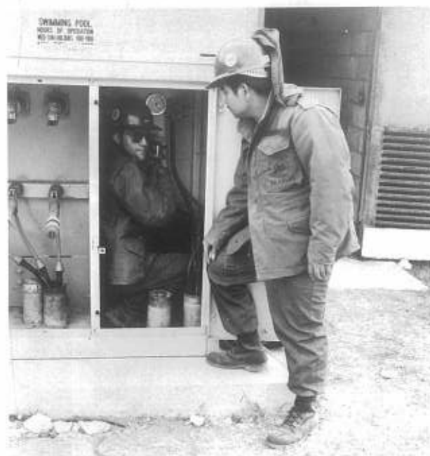
CECA Harmon and CE2 Vinluan hook-up new power lines to swimming pool equipment.
