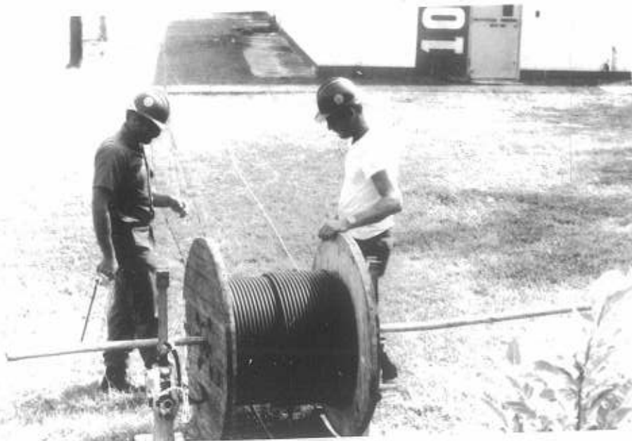
CE3 Avery and CE2 Davis peel cable off reel prior to cutting to length and hanging.
