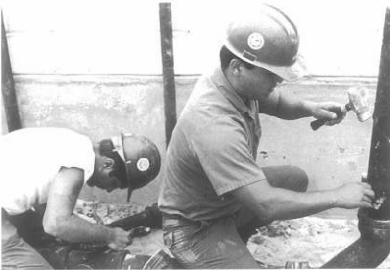
UTCN Gonzales and UTCN Sheppard place packing in connections prior to leading.
