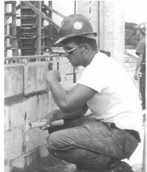
BUCR Rennison and BU2 Doyon jitterbugging and filling voids in concrete work.
