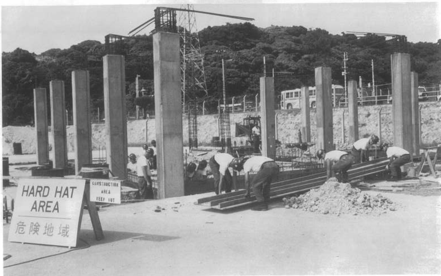
The Pesticide storage crew sets forms for the footer.
