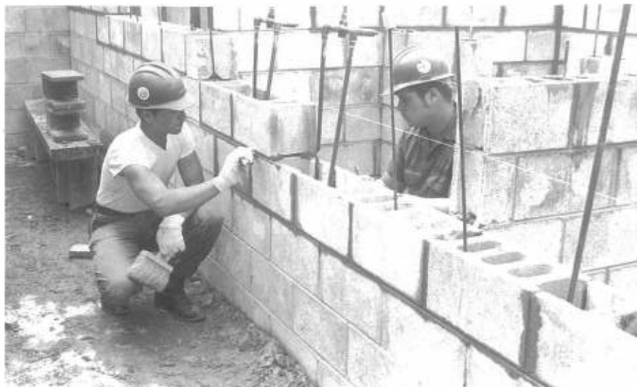
BUCN Lawrence and BUCN Reams lay block and strike joints.
