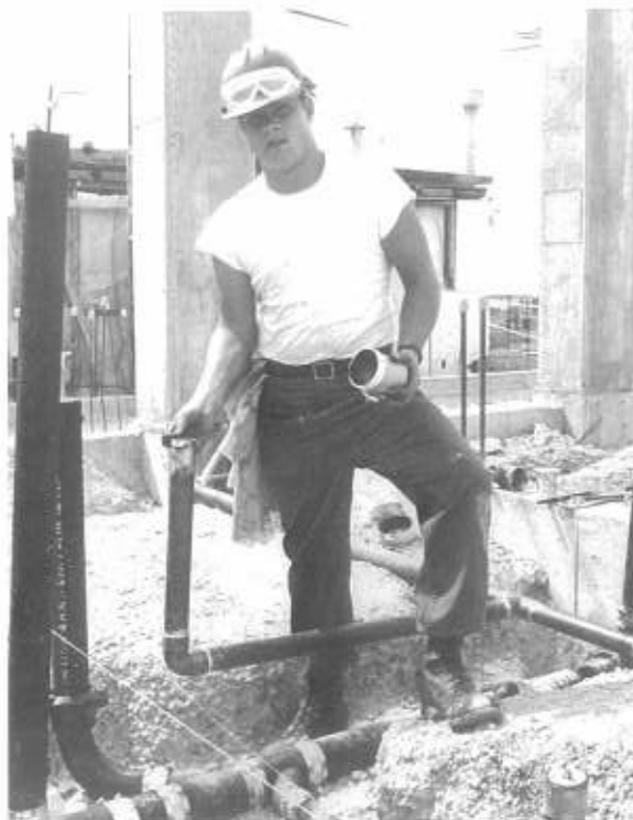
UTCA Beyer fluxes copper pipe prior to soldering.
