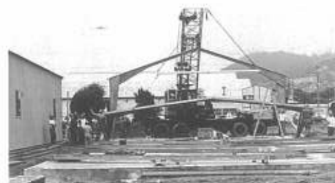
Setting girders at PW Storage
