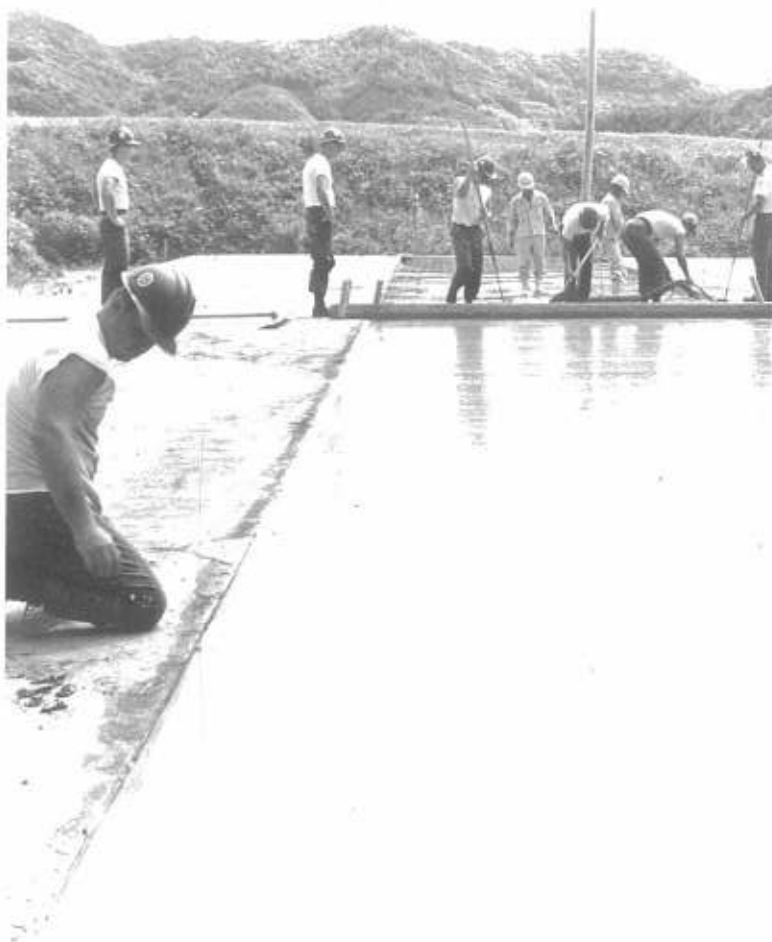
Placing concrete pad for PEB in Hario-Shima area
