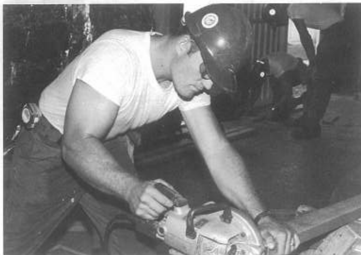
BUCA Kunzie cuts studs for framing for the S-2 remodel.
