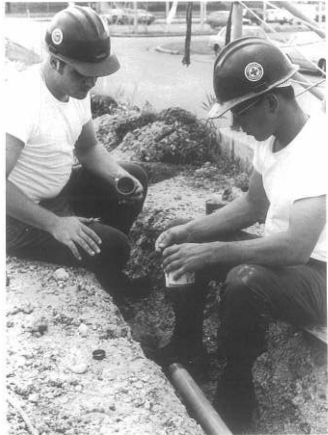
UTCA Arnold and UTCA Greynolds glue plastic pipe for drain at T-350 job site.
