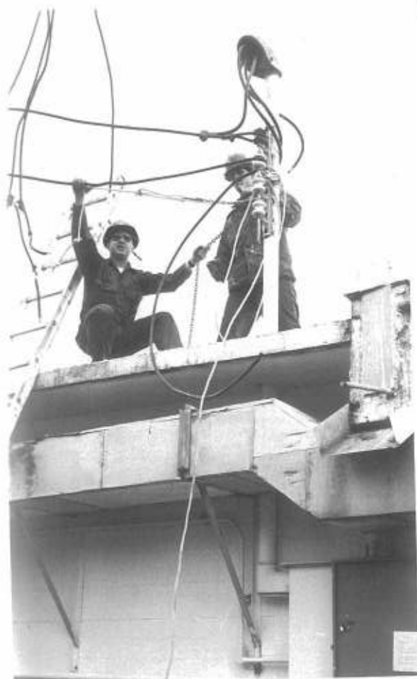
CE3 Billings and CE3 Cassidy pull cable closer to secondary rack on weatherhead.
