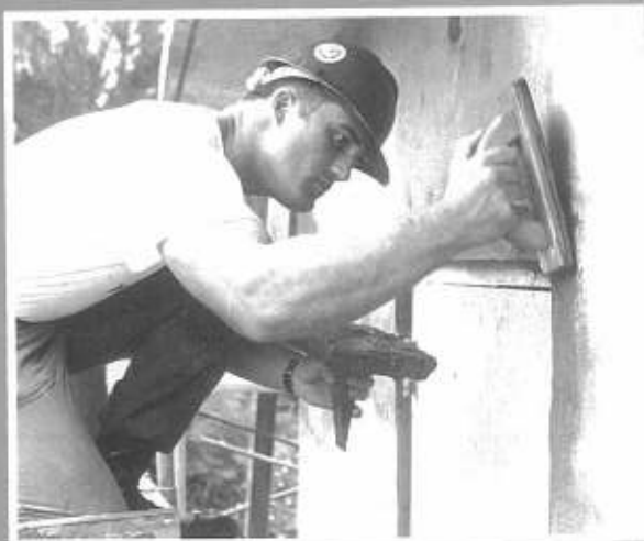
BUCA Kunzie grouting door jam to the tear gas chamber at Camp Schwab.
