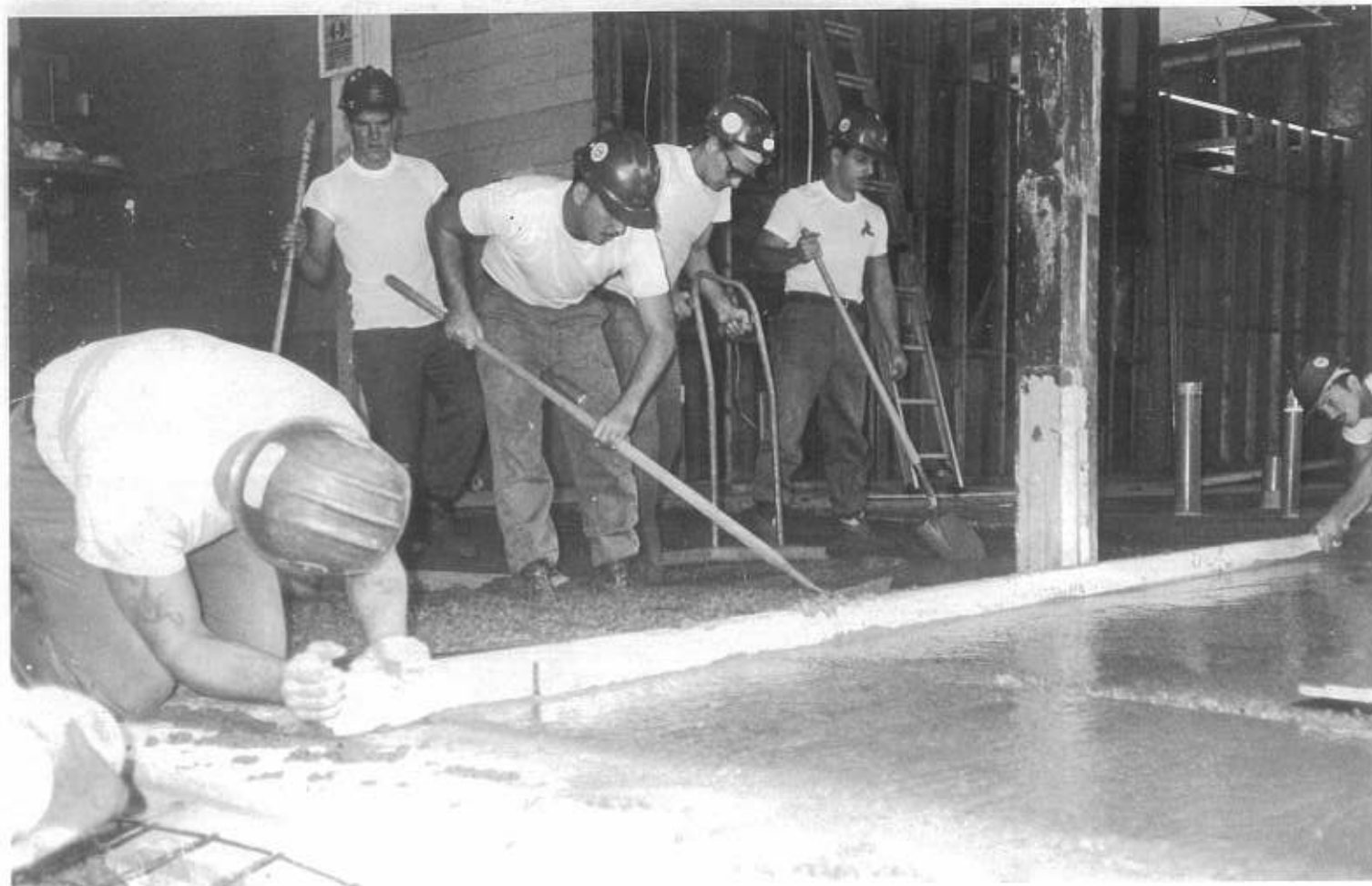
A new concrete floor goes into the renovation of the base gym in Sasebo. Work is being done by the crew of BU3 Gove, BU3 Miller, CE3 Smith, CE3 Kintzer, BUCN Mushaw and BUCN Coffin.
