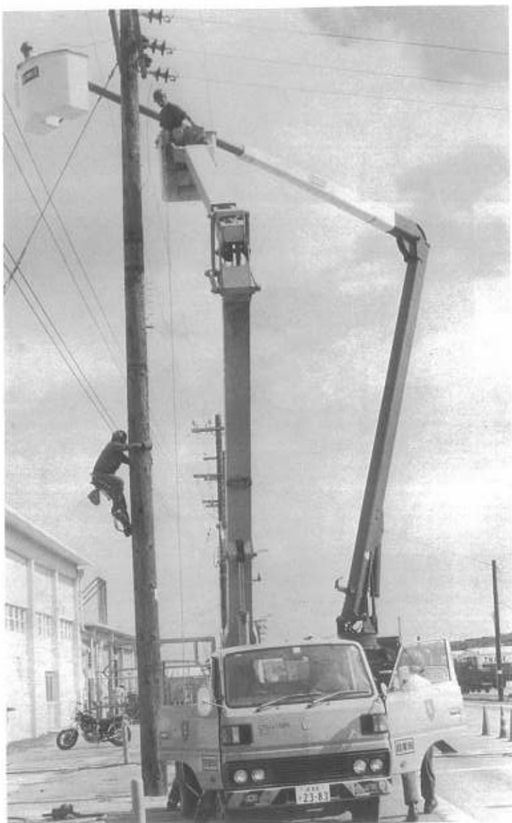
Cleaning the pole prior to removal on the Futenma project.
