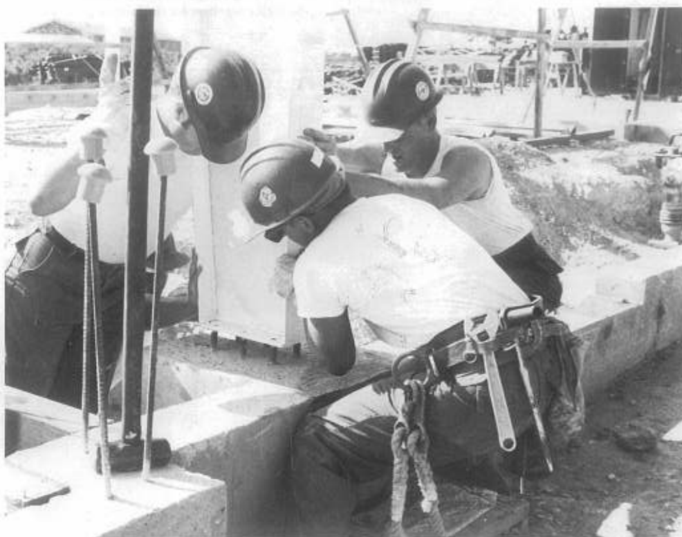
Attaching columns to footer
