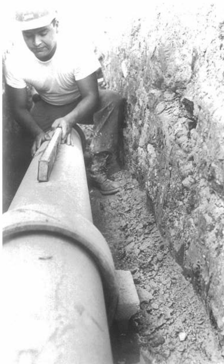
UTCN Gonzales checks fall of drain line.
