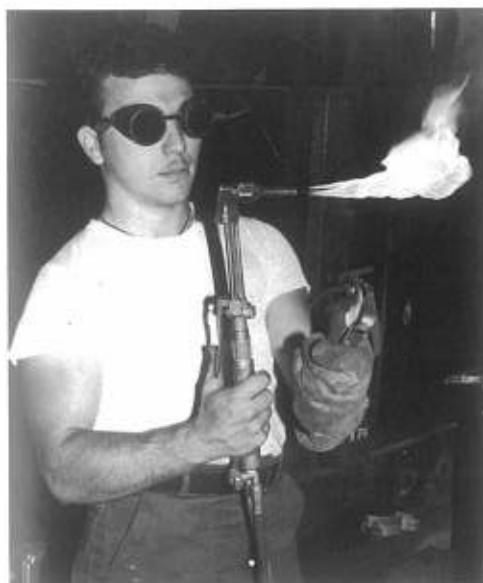
SW3 Balducci lights off a cutting torch.
