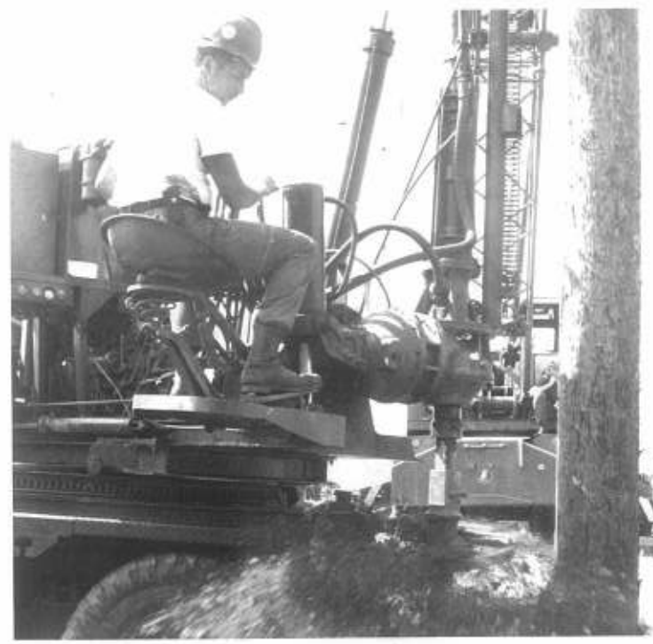
CE2 Lewis operates an auger truck in removal of pole 48A at Futenma MCAS.
