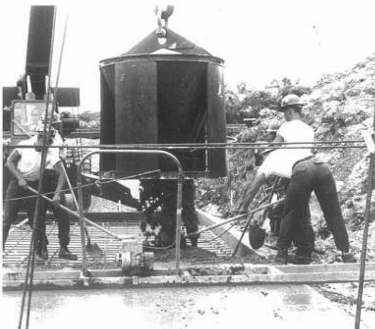
Crew placing footer slab for 60 inch colvert tubes.
