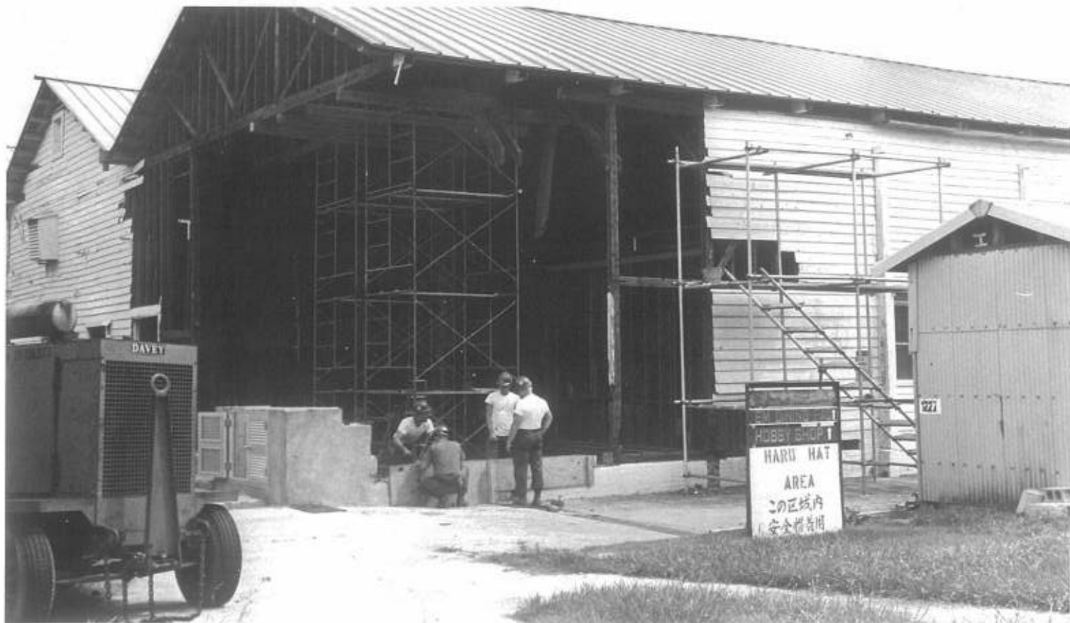
Above — Forming work in progress to raise headwall.
