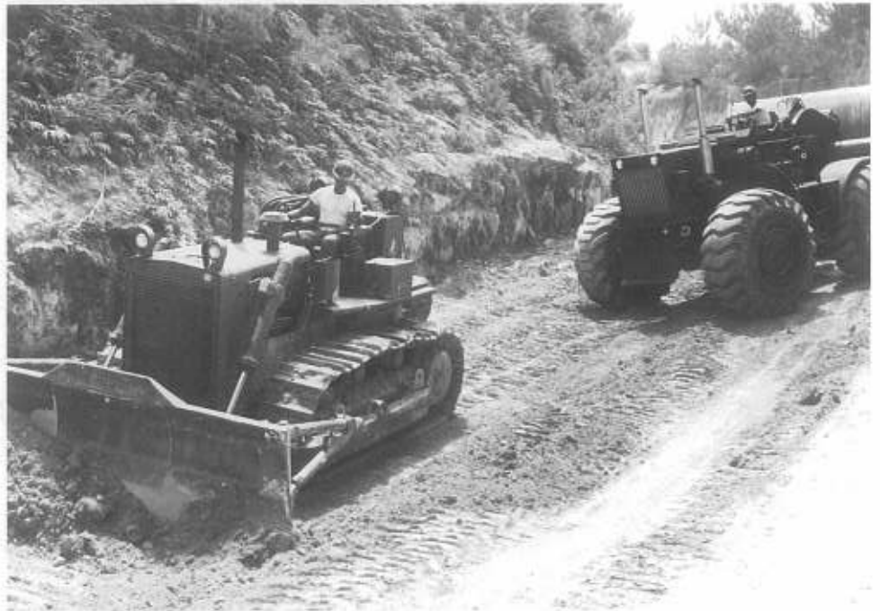
EO3 Wingate on MRS Scraper picking up load broken loose by EO2 Marotta with TD-20 dozer.
