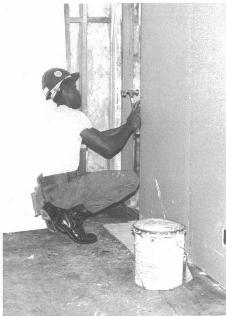
BUCA Keys installs drywall in the new S-2 Office area.
