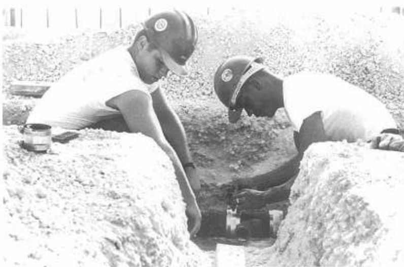
UTCA Beyer and UT3 Brantley clamp down short "ell" connection in steel pipe.
