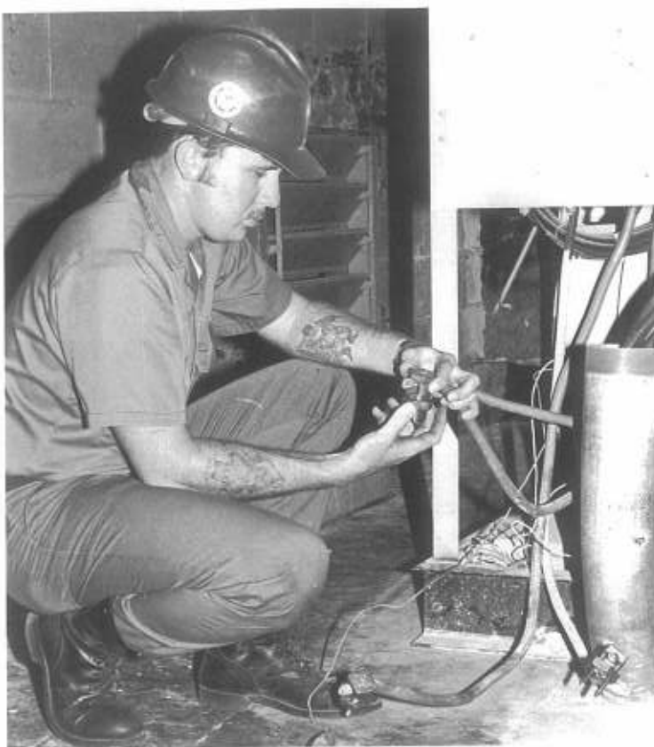
CECN Barnett hooks-up 88KW generator for emergency power.
