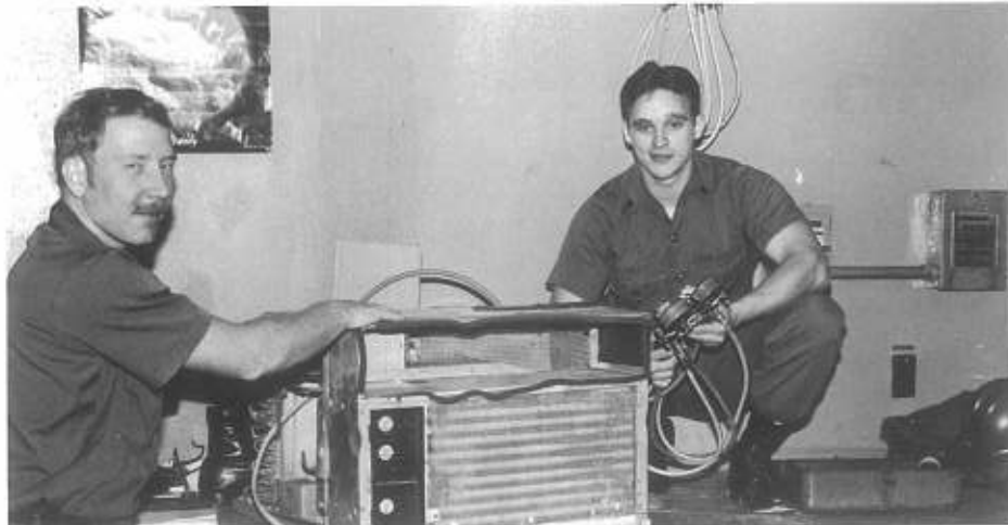
Above — UT2 Fouts and UT3 Yingst check pressure in A/C unit.
