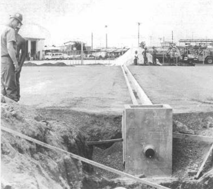
Trench for the oil/water separator in the drum storage lot
