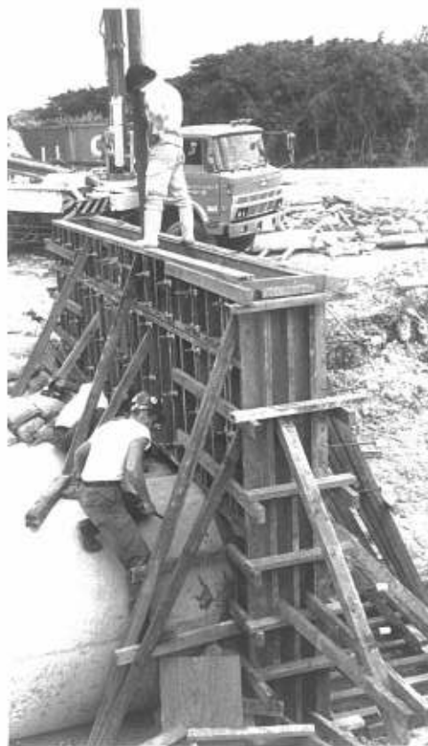
Crew placing footer slab for 60 inch colvert tubes.
