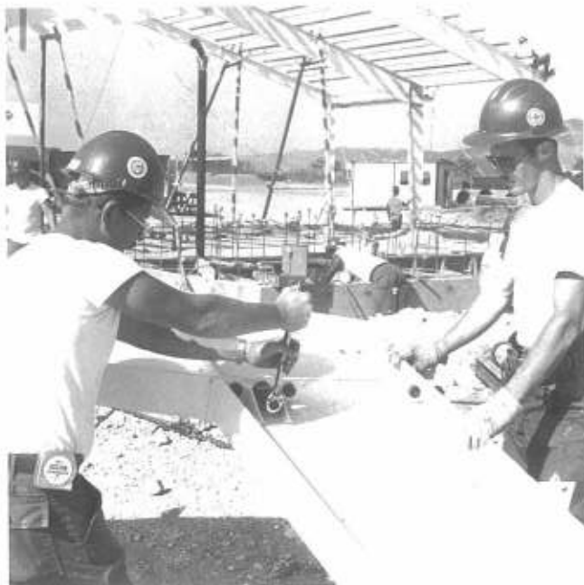
Above — BU1 Bell and SW3 Faiola bolt the rafters together for the Bulter Building.
