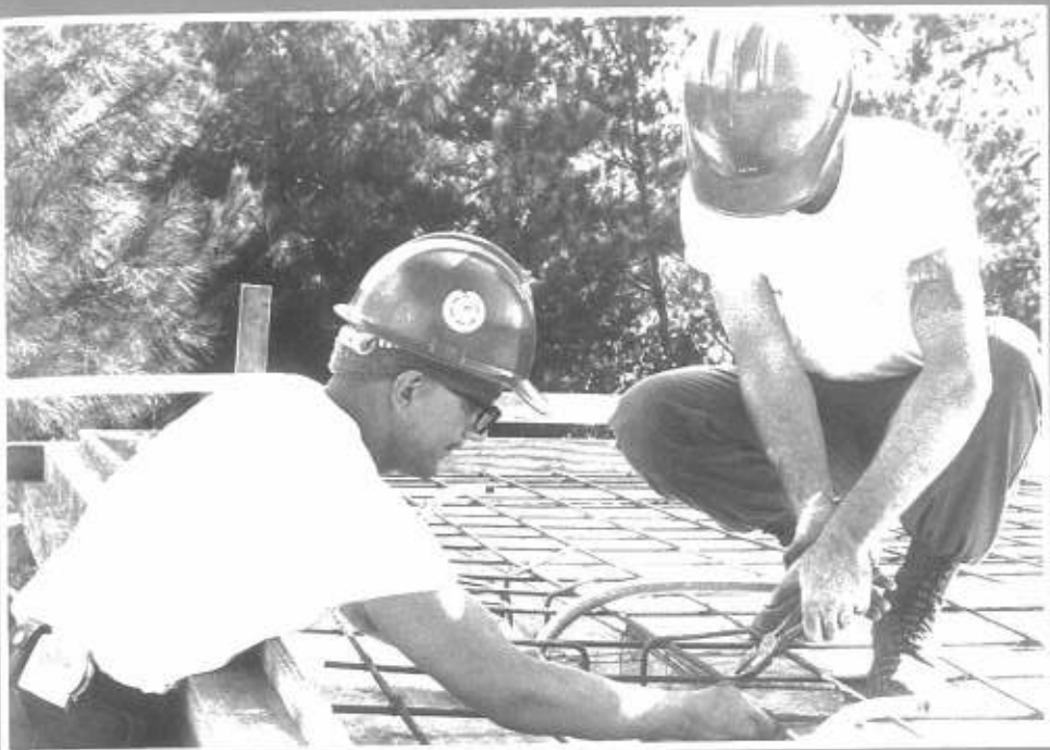
BU2 Debellis and BUCA Keys tie rebar for the roof of the tear gas chamber at Camp Schwab.
