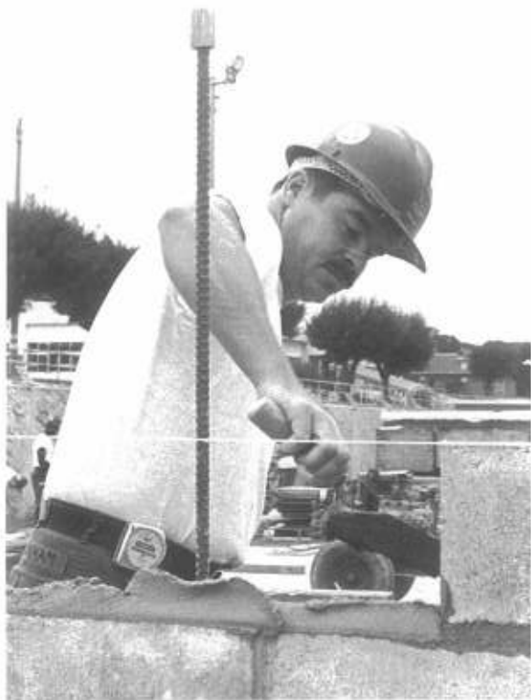
BU2 Dunham places mortar to set block.
