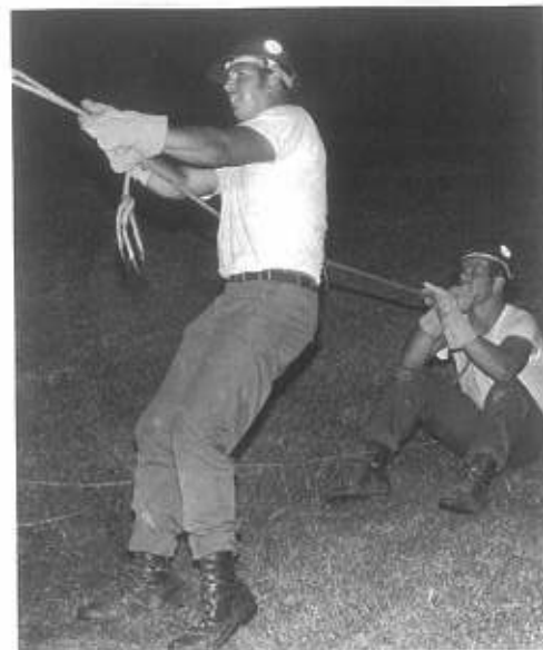
CE1 Patnaude and CECN Carpenter apply tension to guide wire prior to pole removal.
