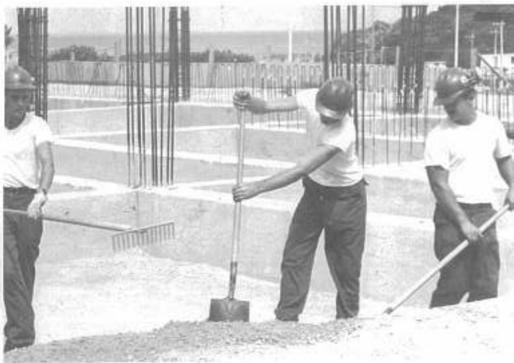
Back filling around the footers at T-350.
