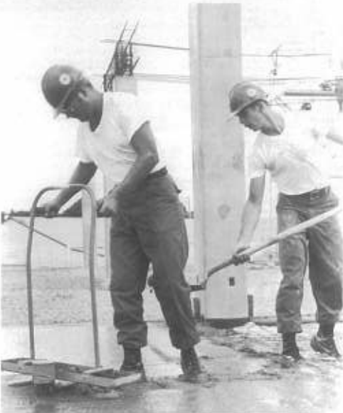
BUCR Rennison and BU2 Doyon jitterbugging and filling voids in concrete work.
