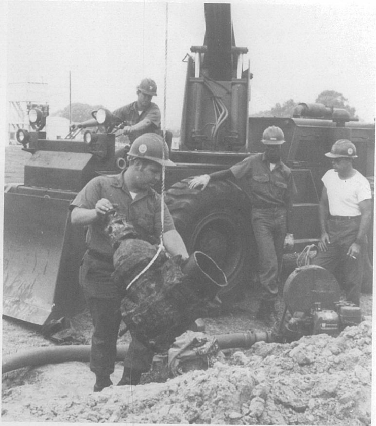
Removing one of the eight inch valve was only a small part of the entire job.
