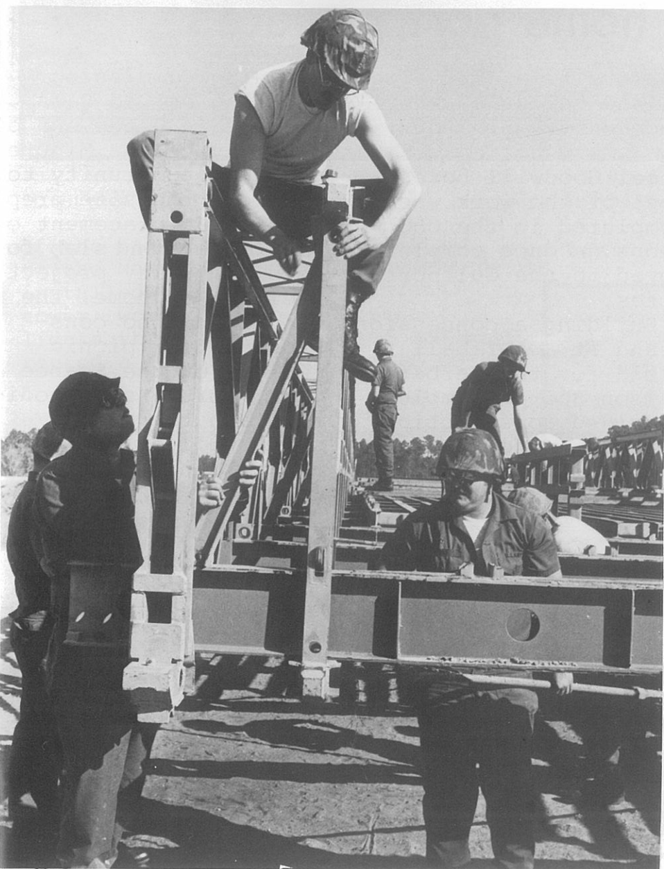
As part of the readiness training, the Minutemen practice building a Bailey bridge.
