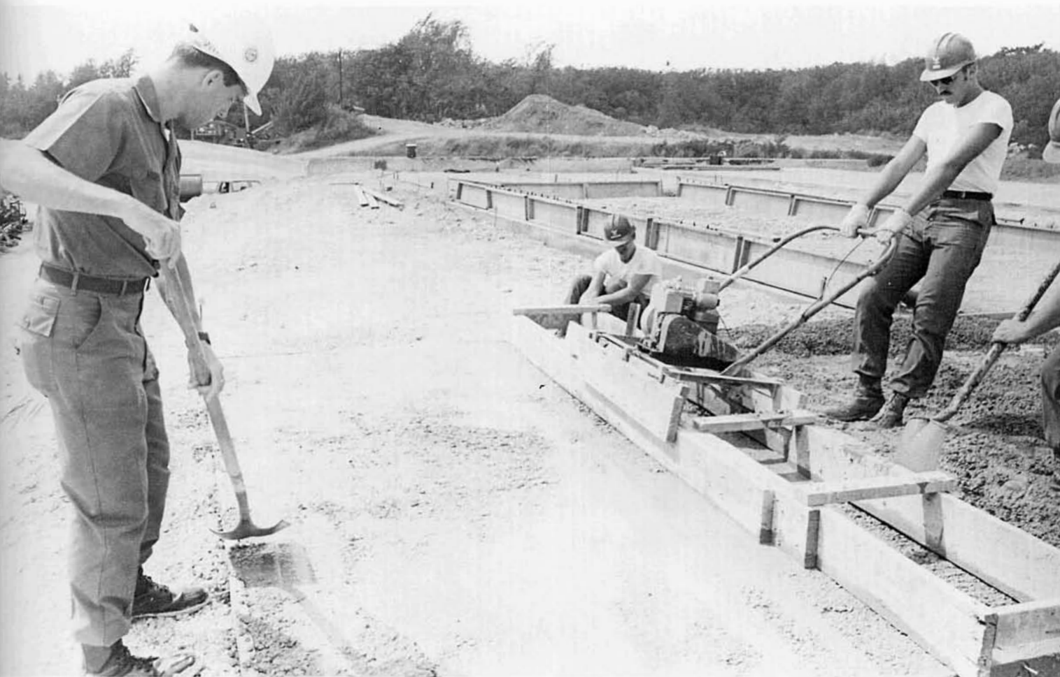
LT Gary Hobson, BU3 Charles Schintzius and BU3 Jeffrey Spier smooth concrete after a pour at the Asphalt Plant.
