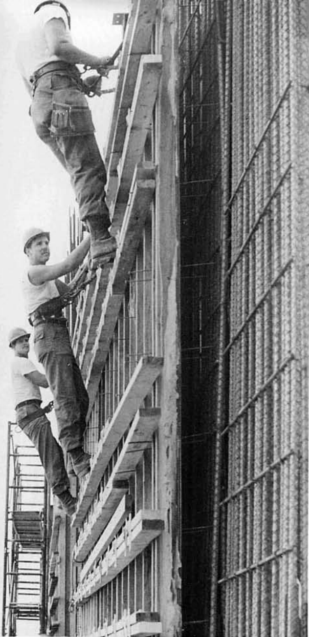
BUCA Jamie Richards, BU3 Mike Saam and another Minuteman prepare a wall for a concrete pour.
