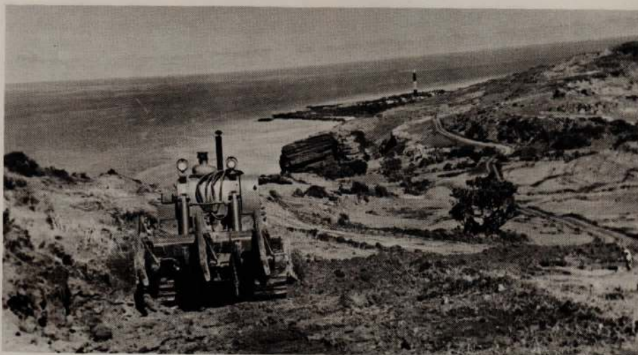
A ROAD AND A PIER -- (Above) Using a TD-20 dozer to do the job, an equipment operator carves a road up the steep volcanic slope on Cu Lao Re Island. (Below) Steelworkers on the shore fabricate the pier to be used for unloading supplies. In the background a group of islanders stand watching.
