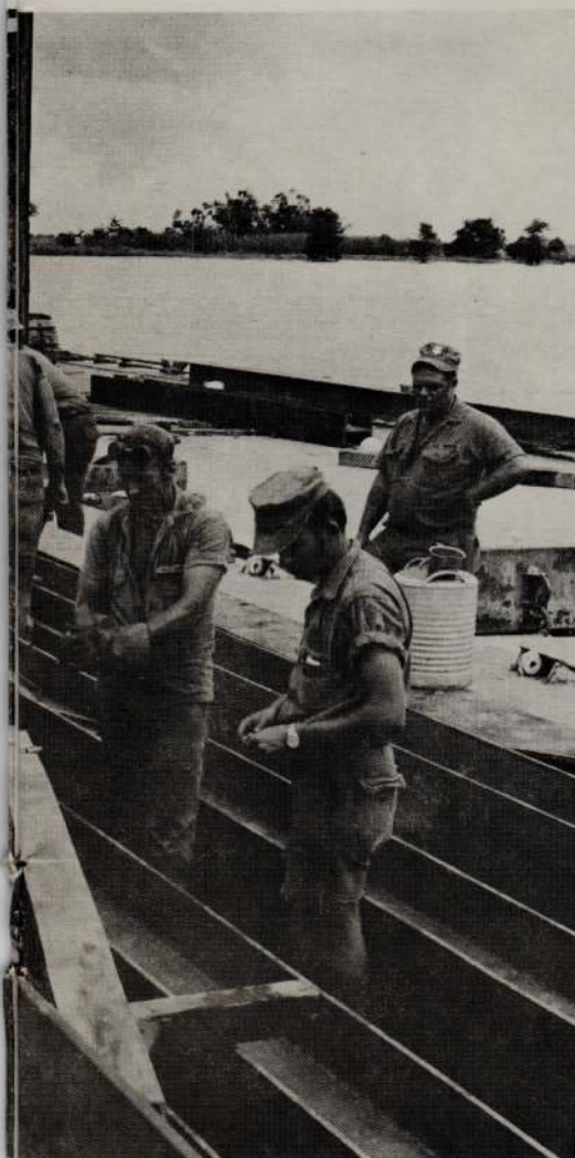
STEEL TO GO DOWN -- (Bottom) Steelworkers at Albany's site are busy with construction of the pontoon pier. The steel wide-flange sections are used as piles to which are secured the pier.
