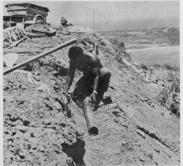
UTILITIES MAN THIRD CLASS RALPH COPELAND places a section of sewer pipe in place at the Observation Point. This was part of the task of upgrading the site for men who must live there during firing exercises.
