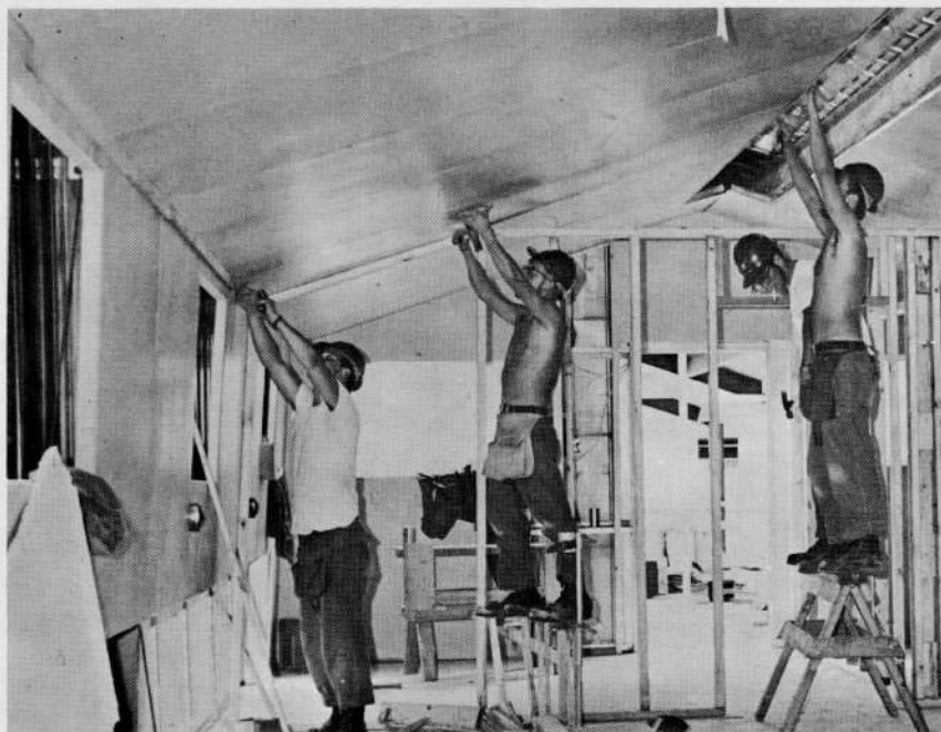
GETTING IN OVERHEAD--Seabees of Detail Guantanamo install a ceiling in a berthing hut for Marines on Camp Bulkeley aboard the Naval Base, Guantanamo Bay, Cuba.
