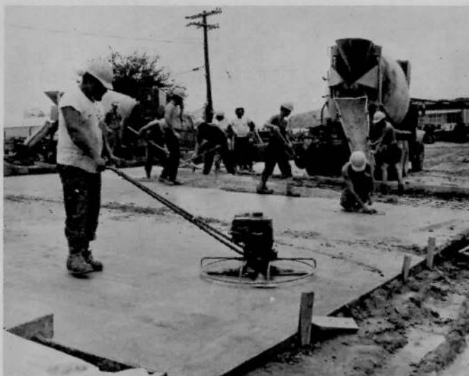
DELTA COMPANY PERSONNEL work on concrete slab for a new vehicle wash rack in the Alpha Company yard.
