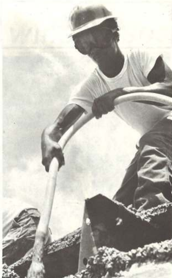
Worker at the NavMag theatre project uses a vibrator to release air bubbles trapped inside freshly-placed concrete.
