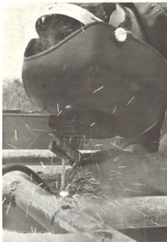
Seabee arc-welds steel tubing that makes up framework of Echo company's flotation barge for the Lima Wharf project.
