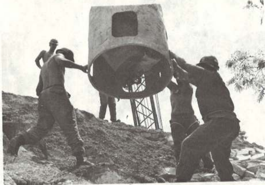
E0CN J.D. Clark, E02 Ted Seaton and E02 James O'Neal strain to position a bucket loaded with cement grout for placement over a section of concrete rip-rap.
