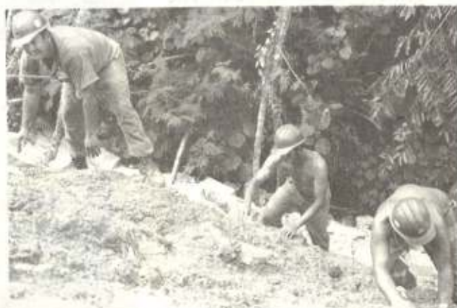
Mountaineering Seabees make their way up the steep grade, hand-forming freshly-placed grout over rip-rap, ensuring a good seal. (photos by JO2 PM Callaghan)
