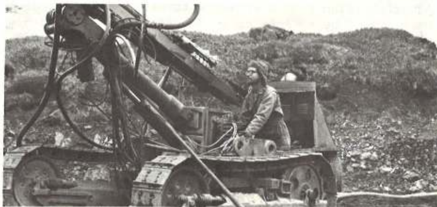
E02 Mike "Powder Monkey" Bowen works rock drill in spite of Adak's cold winds to blast rock for the Zeto Point seawall project. (Official US Navy photo)
