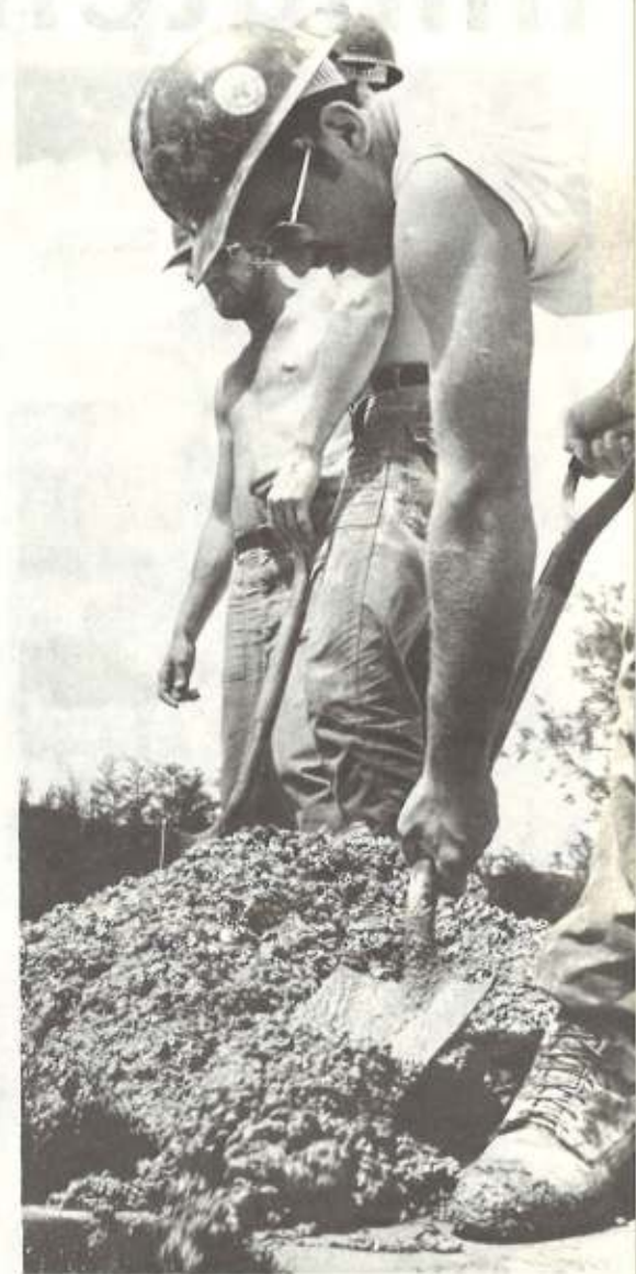
ABOVE: As the concrete bucket moves away for refilling, BU3 Tony Krant shovels concrete into wooden forms for the theater wall. (photo by JO2 Callaghan) LEFT: After four months of el-
